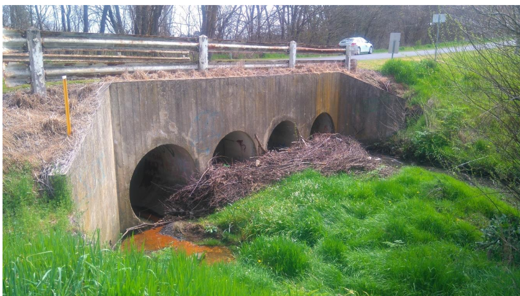
Figure 4-40 Blockage at the Ebdon Street culverts
