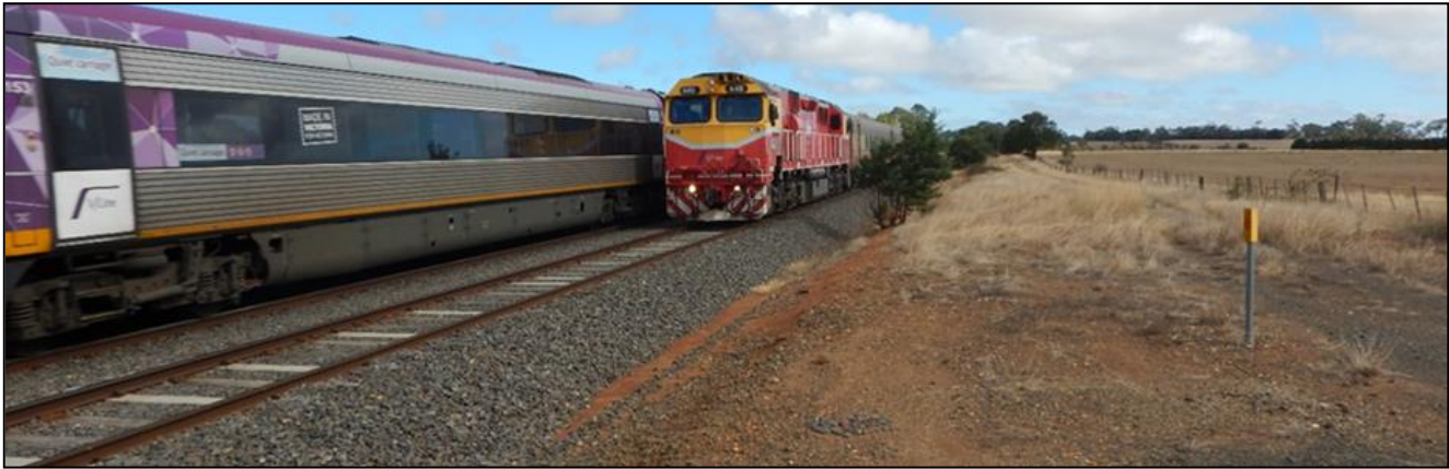
IMAGE 7 - THE CLOSE PROXIMITY TO THE RAIL AND SEVERAL ROAD RAIL CROSSINGS MAKES THE ACTIVE RAIL CORRIDOR LESS APPEALING TO WOODEND.
