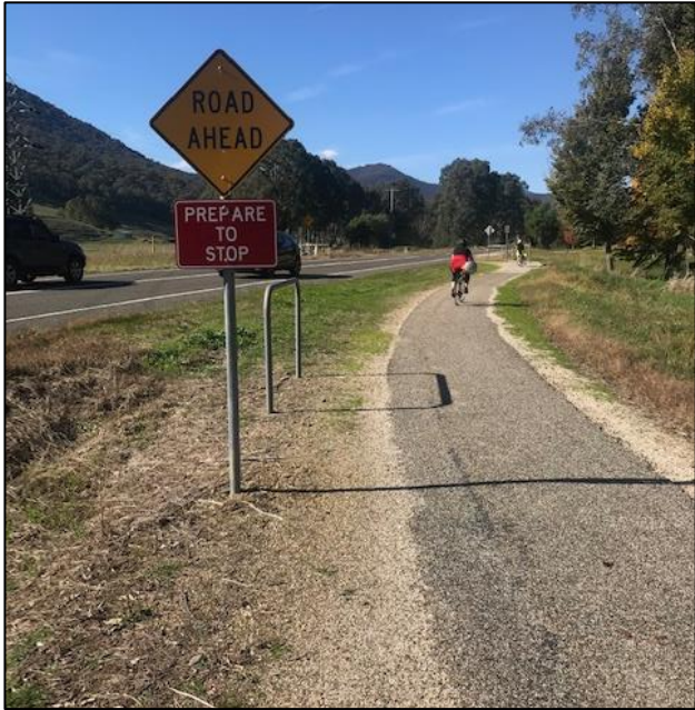
IMAGE 11 - ROAD CROSSING TREATMENT (MURRAY TO MOUNTAINS TRAIL)
