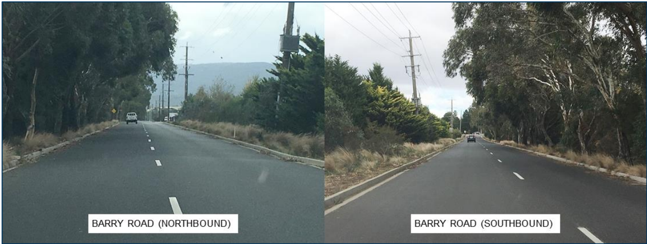
Figure 2-8 Barry Road South of Ladd Road
