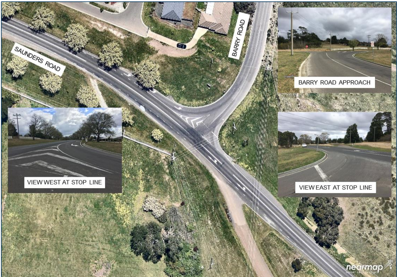
Figure 2-9 Existing Saunders Road / Barry Road Intersection
