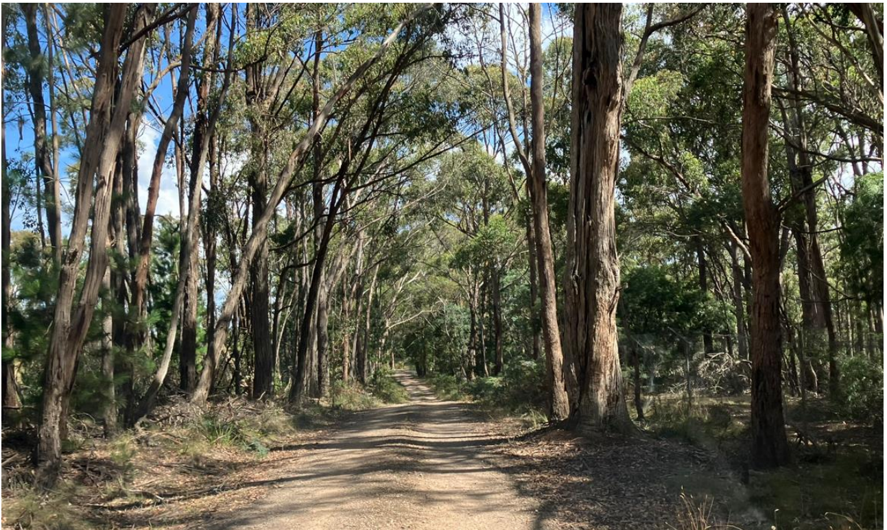
Figure 4 – Emmins Road Existing Condition
