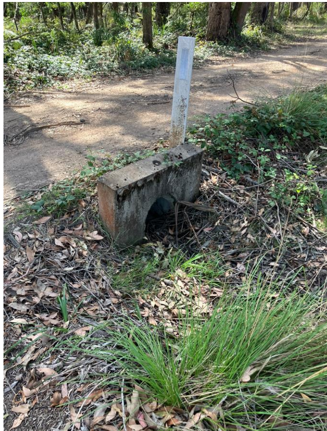
Figure 7 – Existing Pipe Culvert drainage system
