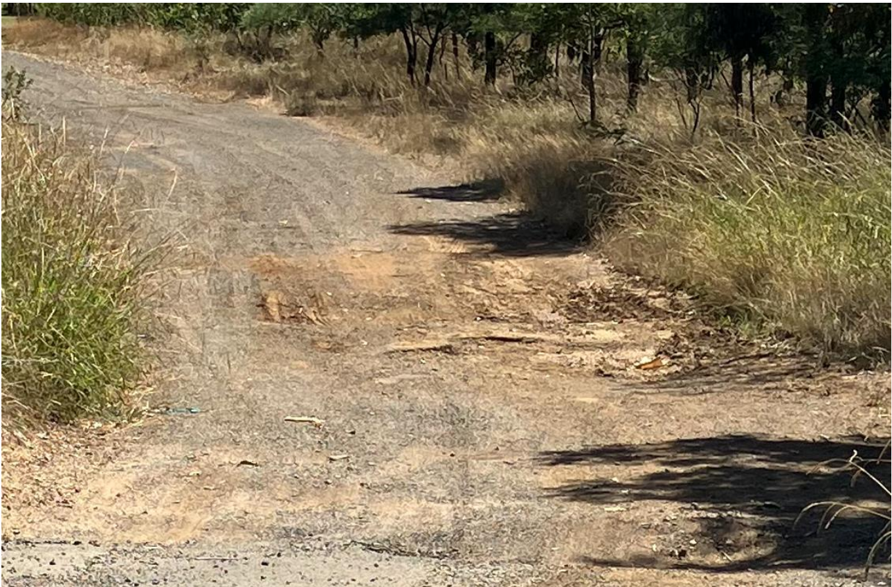
Figure 4 – Existing Pipe Culvert drainage system
