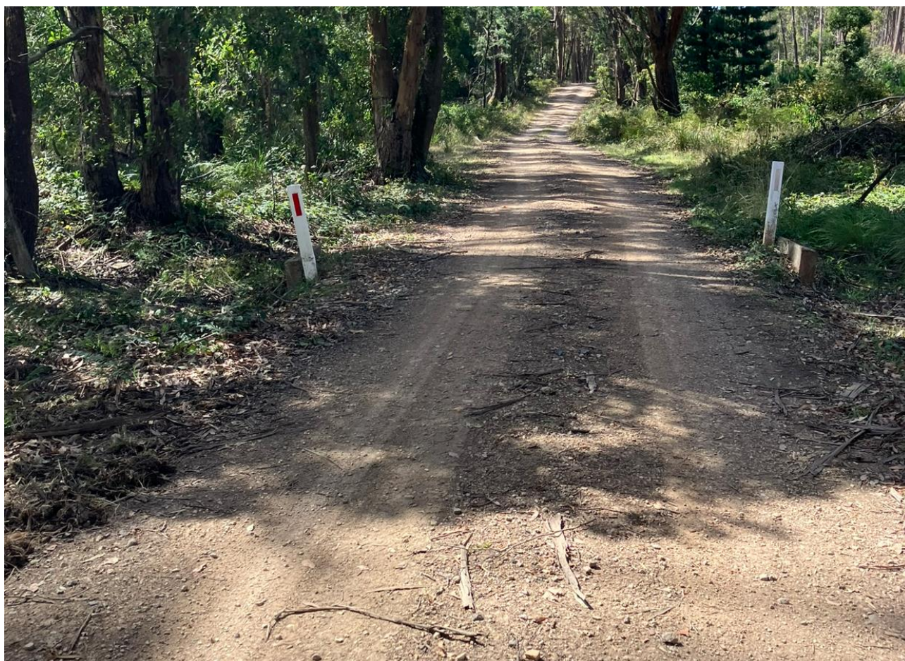
Figure 6 – Typical Potholes
