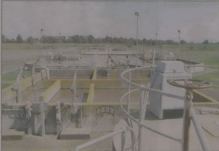
The Kyneton Water Reclamation Plant.
