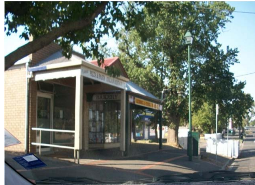
Photo 4.1 Main Road, single storey building
