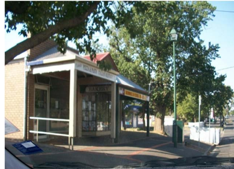
Photo 2.2 Main Road, single storey building
