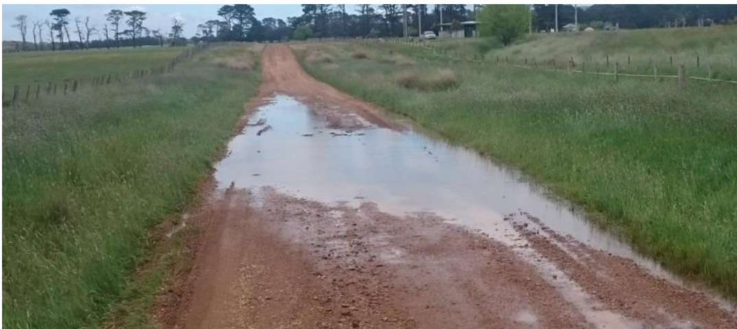
Figure 7 – Ponding 1 of 2
