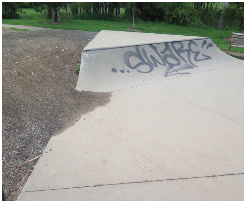
ISSUE: Debris ending up on skatepark SOLUTION: Hardstand area to connecting different areas
