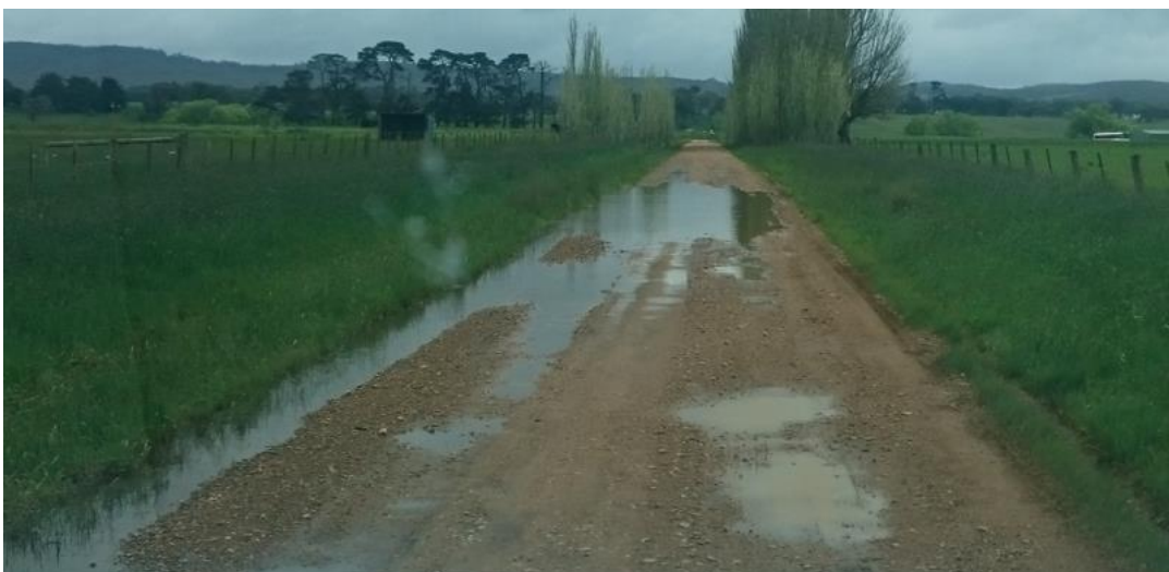
Figure 8 – Ponding 2 of 2
