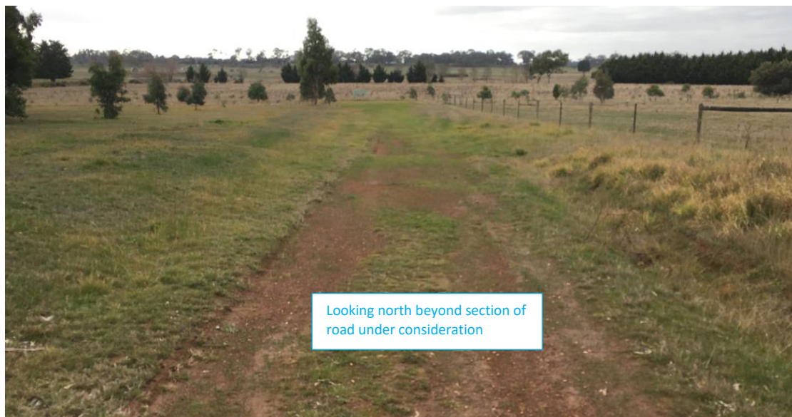
Image 3 – View North of Subject Road Section
