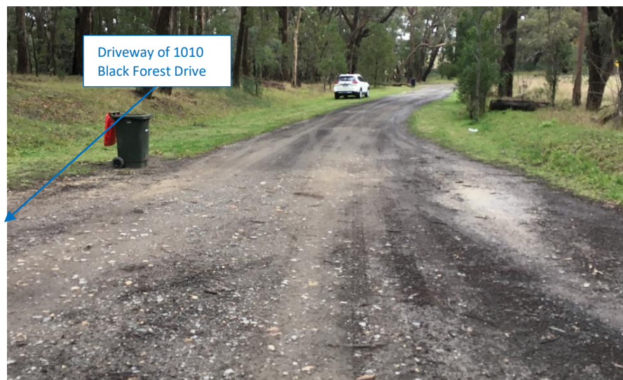
Image 3 – View of Subject Road Adjacent First Driveway
