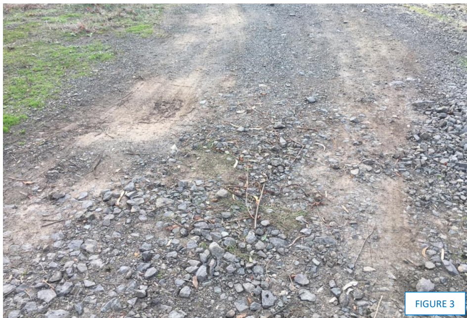
Image 4 – Subject Road, Pot Holes and Surface Damage
