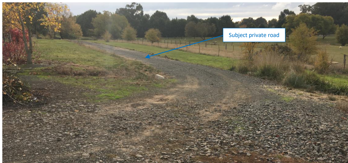
Image 2 – Subject Road Looking North West
