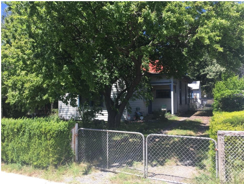
Figure 11. Possible former stationmaster's house
