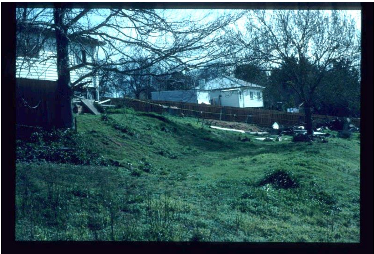
Figure 7. Gisborne Shelter Shed, c.1992 (Heritage Victoria)
