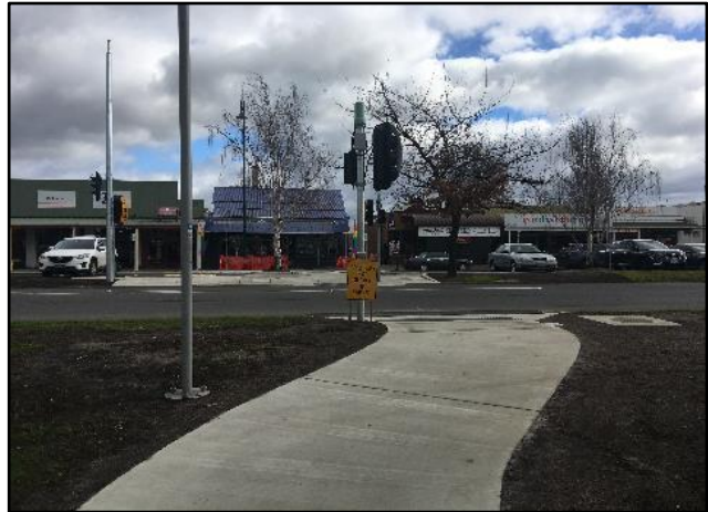
Figure 3-30 New Signalised Pedestrian Crossing on Aitken St
