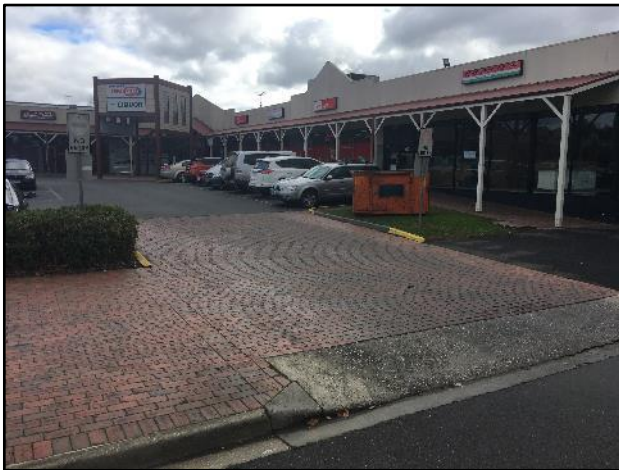
Figure 3-32 IGA Car Park Crossover on Brantome St
