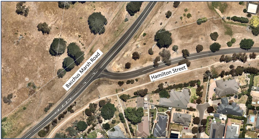
Figure 5-10 Existing Bacchus Marsh Road / Hamilton Street Intersection
