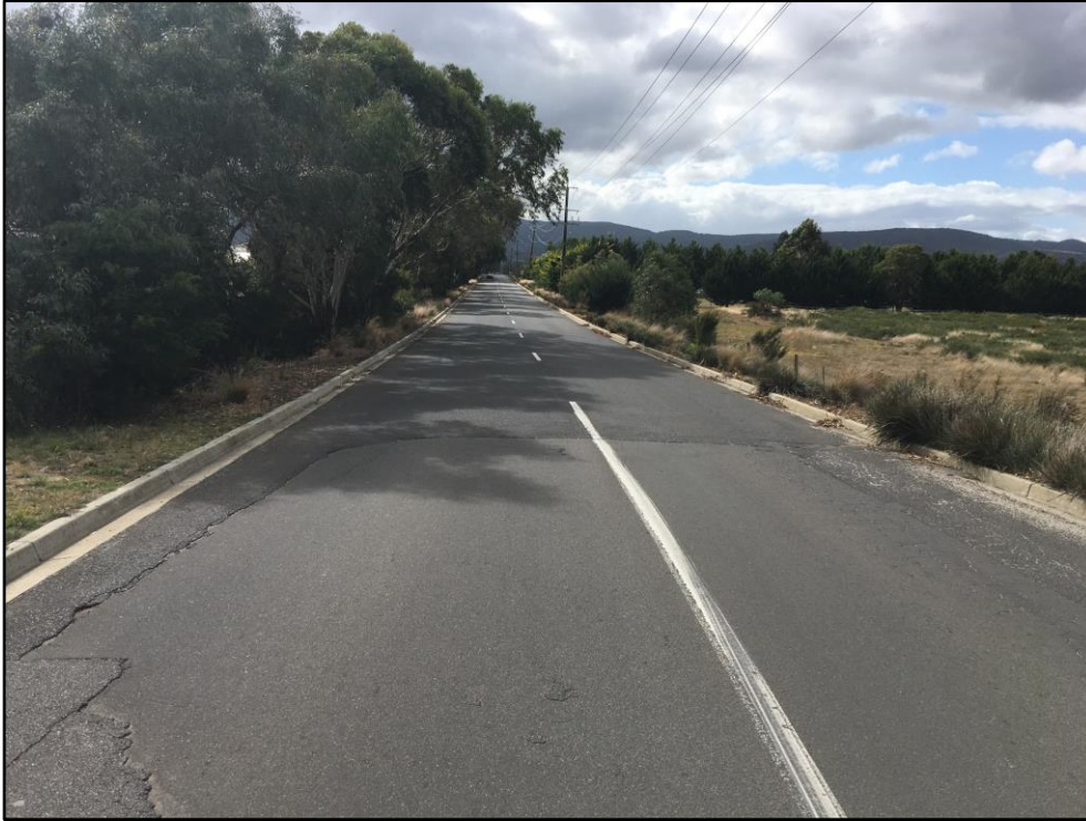
Figure 3-16 Barry Road Northbound from Saunders Road
