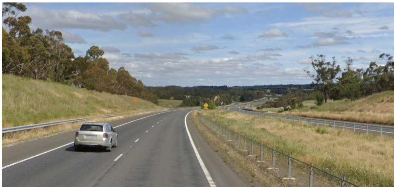
Figure 3-5 Calder Freeway Southbound, near Kilmore Road Overpass
