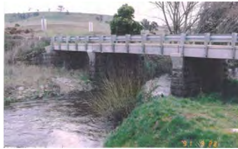
Figures 13 & 14. Bluestone (L) Culvert Abutments over Limbricks Creek, Morris Lane, Pipers Creek (HO183) (R) Manning's Bridge, Springhill Road, Spring Hill, 19th century substructure with later road deck (HO232) (Source: D Bick et al, Kyneton Conservation Heritage Study, vol 7, 1990)
