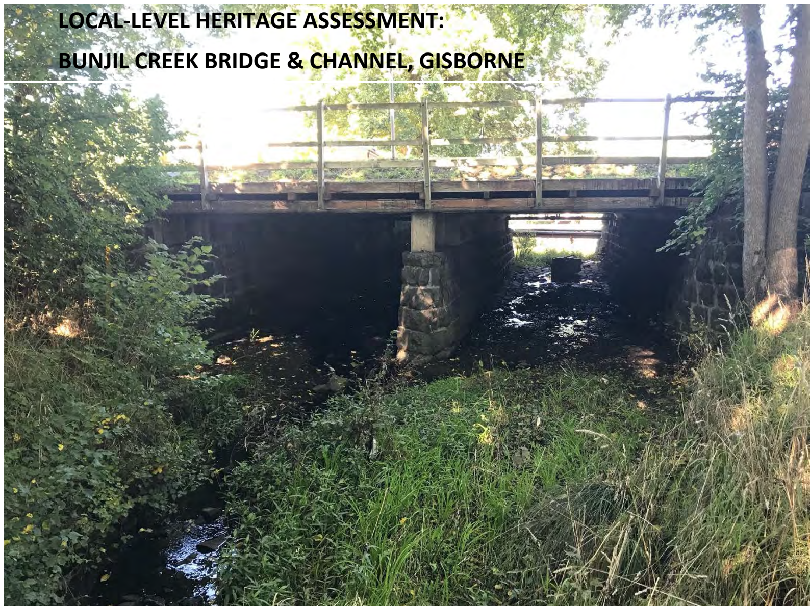
Figure 1: Bunjil Creek Bridge & Channel (GJM Heritage, March 2020)
