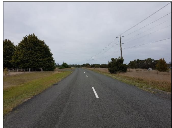
Figure 6: Bennett Road (View South)
