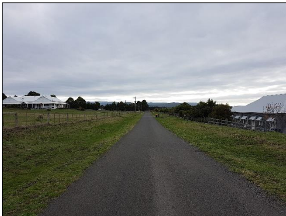
Figure 9: Coney Road (View North)
