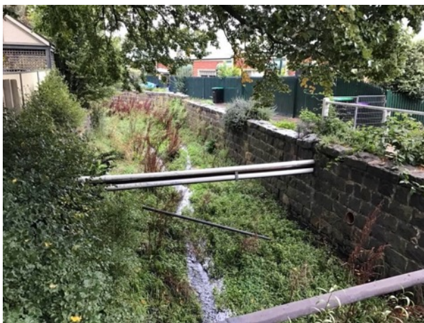
Bluestone rockwork and drains within Bunjil Creek.
