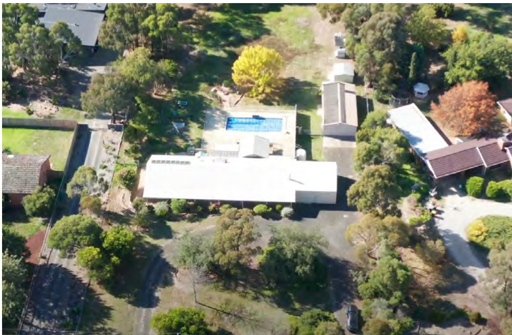
Figure 3 – Subject site from Richardson Street (aerial view)
