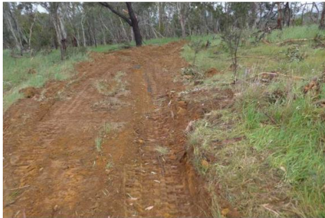
Grading for drainage lines. Photo: Newham Landcare
