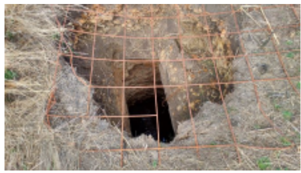
Image 3. Bore hole in the north of the property still supporting water (Abzeco 24/03/2020).
