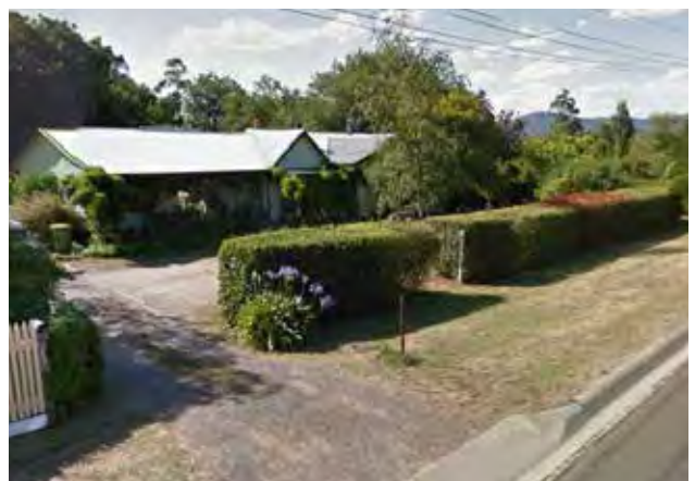
Photo 6. Precinct 1b: Station Road
