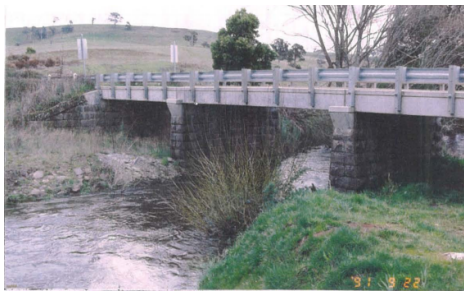
Figures 13 & 14. Bluestone (L) Culvert Abutments over Limbricks Creek, Morris Lane, Pipers Creek (HO183) (R) Manning's Bridge, Springhill Road, Spring Hill, 19th century substructure with later road deck (HO232) (Source: D Bick et al, Kyneton Conservation Heritage Study, vol 7, 1990)
