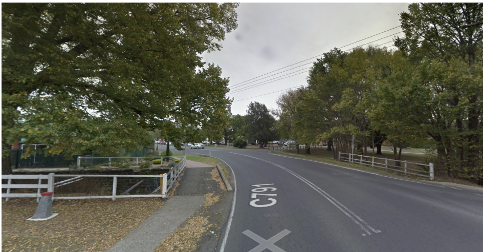
Figure 7. Approach to the Bunjil Creek Bridge from the south. (Source: Google Maps May 2018)
