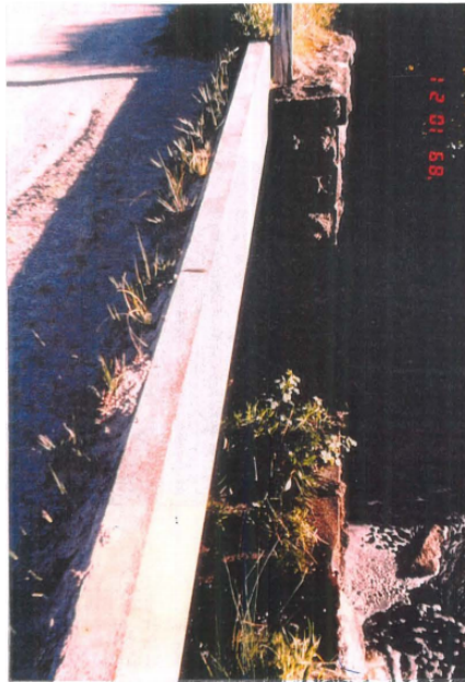
Figures 11 & 12. (L) Stone Bridge Abutments and Piers, Hodges Bridge, Boundary Road, Edgecombe (HO20), Note: 20th century timber deck and balustrade (R) Bluestone Road Bridge Abutments, Central Road, Kyneton South (HO47) (Source: D Bick et al, Kyneton Conservation Heritage Study , vol 6, 1990)
