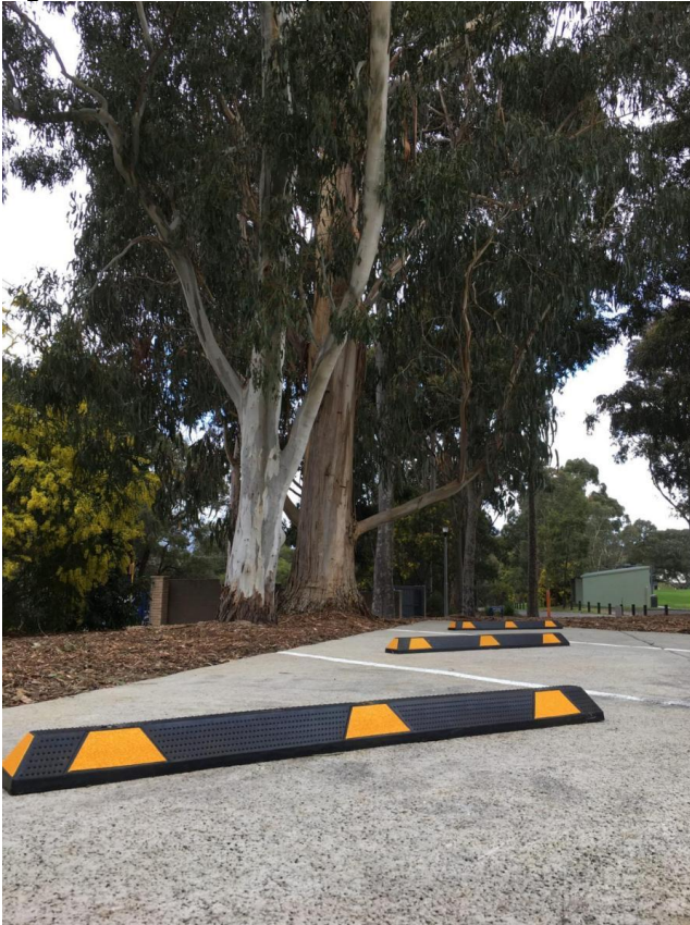
Figure 5. Yarra Valley School RINGWOOD VIC - DriveCon natural
