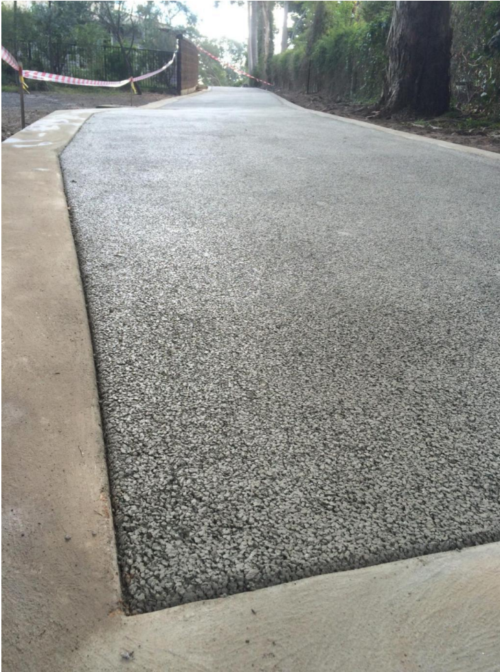
Figure 1. Brysons Road WARRANWOOD VIC - DriveCon with bluestone oxide.
