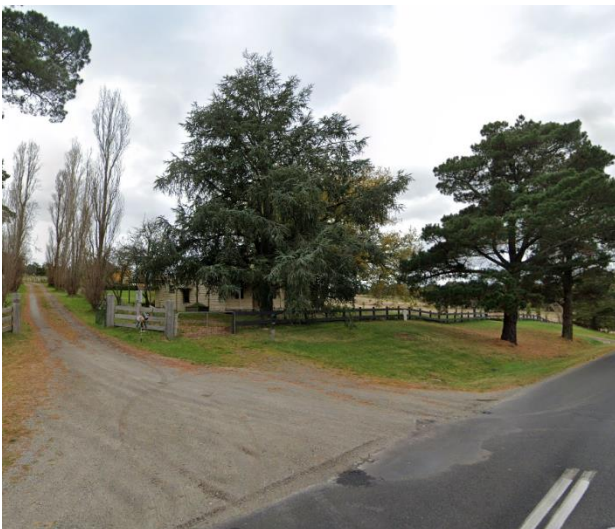
Figure 1 (looking south west - May 2021)
