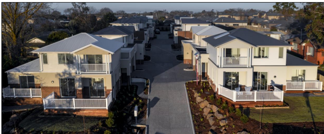
Figure 11: Modern infill dwellings at 27 Calthorpe Street, Gisborne
