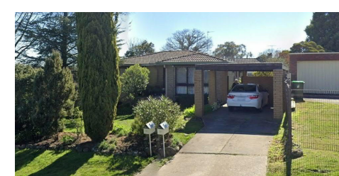
D - 26 HOWEY ST, GISBORNE - VIEW FROM SOUTH
