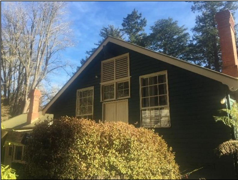
Figure 2. South side of former stables (GJM Heritage/Frontier Heritage, July 2018)
