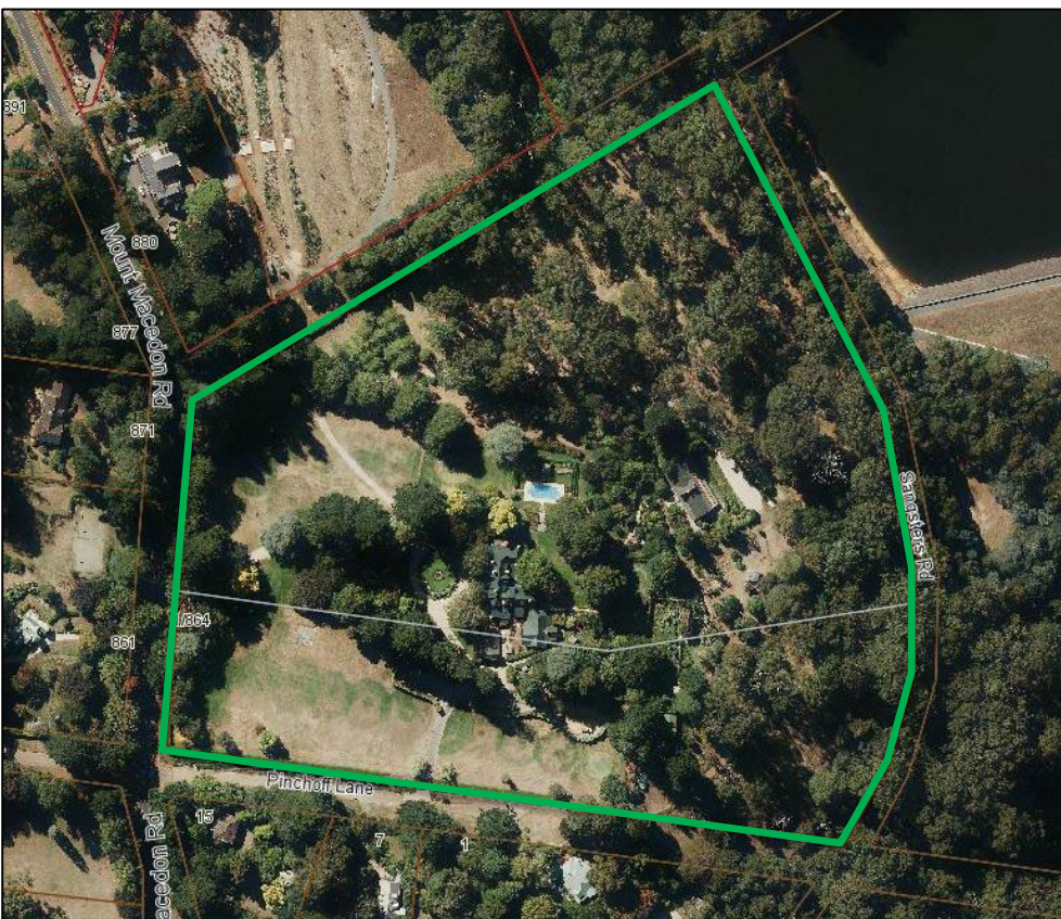
Figure 3. Aerial photo of 864 Mount Macedon Road, Mount Macedon (Source: Macedon Ranges Shire Council, aerial dated March 2018).
