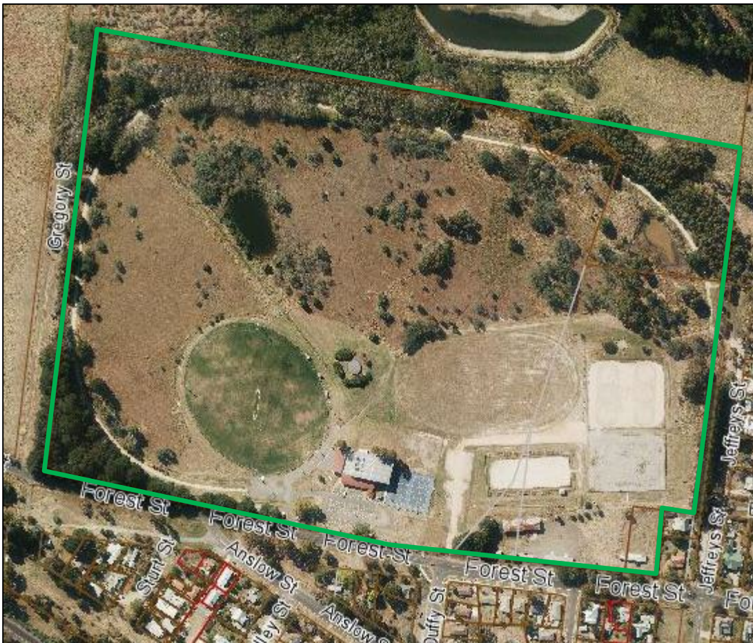
Figure 3. Aerial photo of 1-29 Forest Street and 11 (part) Davy Street, Woodend (Source: Macedon Ranges Shire Council, aerial dated March 2018).
