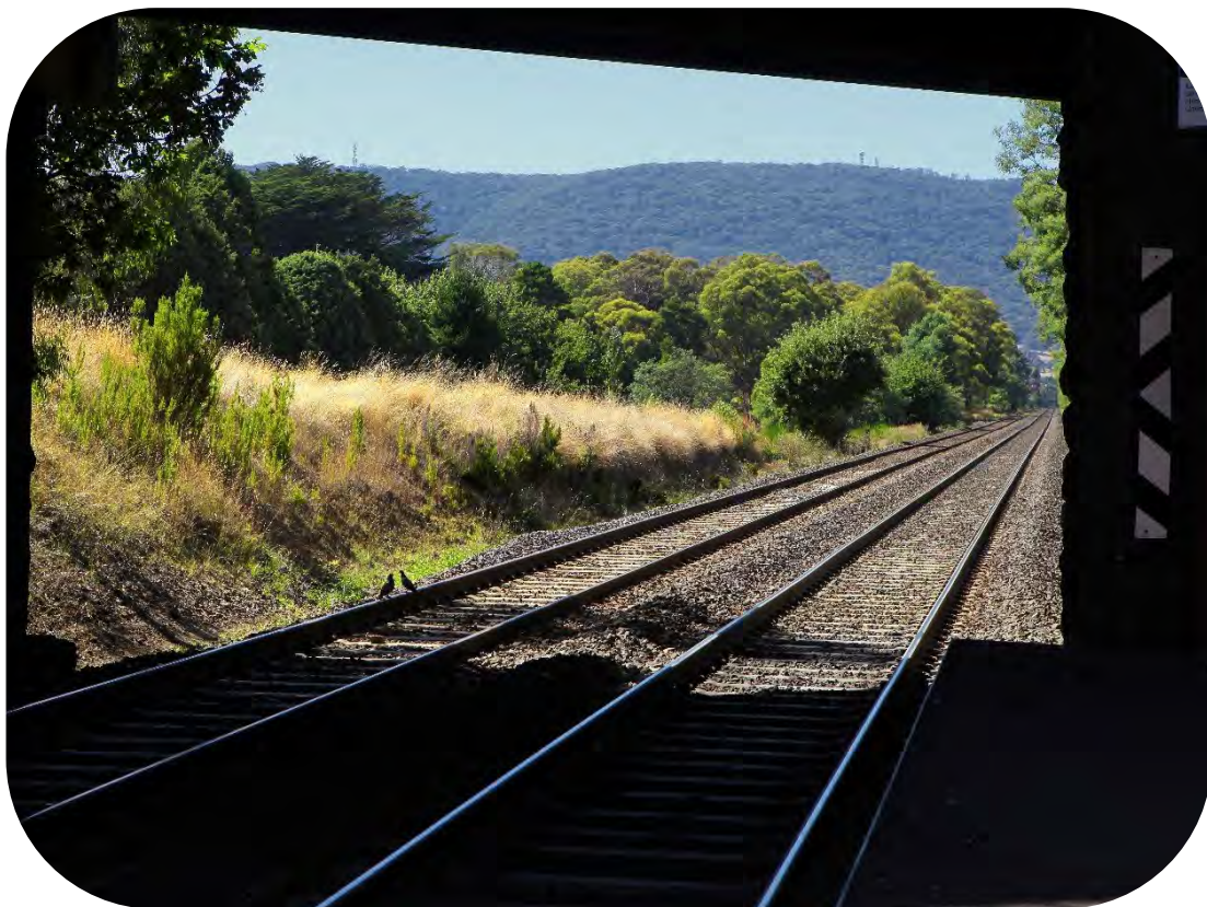
V/Line railway heading towards Woodend Station
