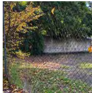
Image 24. Tennis Court hit-up wall, chain mesh fence are unsightly and impede access
