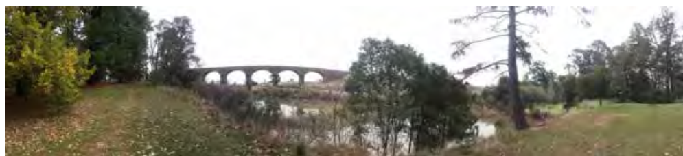
Image 59 : View toward Viaduct from the bank of the Coliban River
