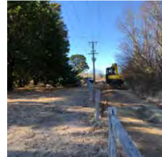
Image 18. Poorly maintained connection to Viaduct and Coliban
