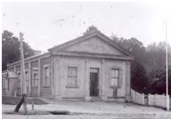
Image 48 c. 1913. The Malsbury Town Hall showing previous timber gate arrangement prior to the Memorial Gate being built. Photograph E. Boddy, Malsbury Historical Society
