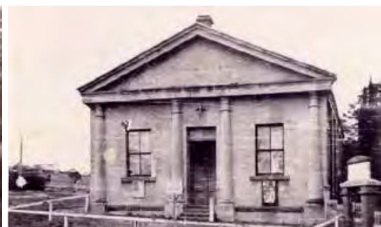
Image 47 Malmsbury Town Hall in 1949 prior to demolition of the façade. State Library of Victoria
