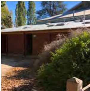
Image 5. Entry dominated by fencing, toilet block and screening shrubs
