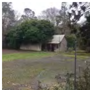
Image 25. Tennis Courts with hit-up wall and pavilion in background
