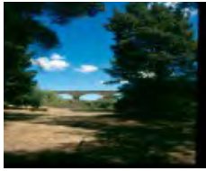
H01993 malmsbury botanic gardens viaduct
