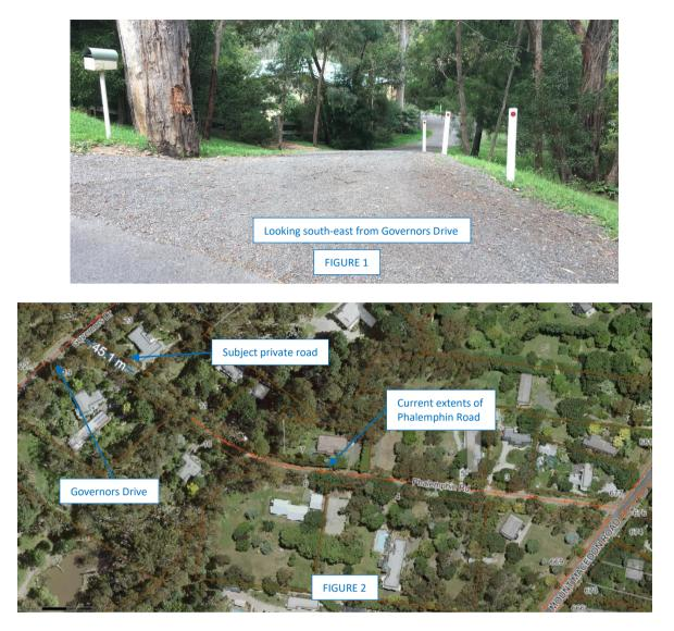
The gravel pavement of the private road is approximately 3m wide and is centrally located within a 15m wide road reserve. Minor loss of gravel material and shape was observed in the pavement.
