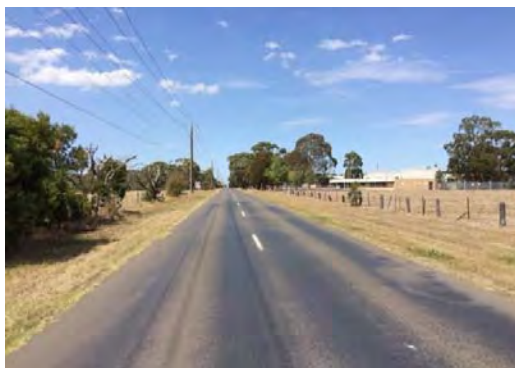
Figure 3-24: Hamilton Road East (looking E)
