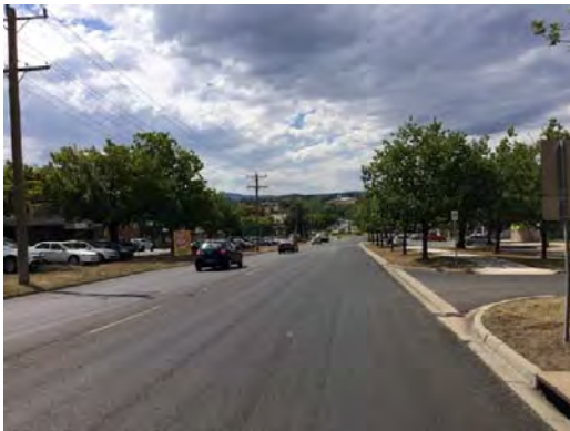
Figure 3-2 Gisborne Melton Road (looking N)
