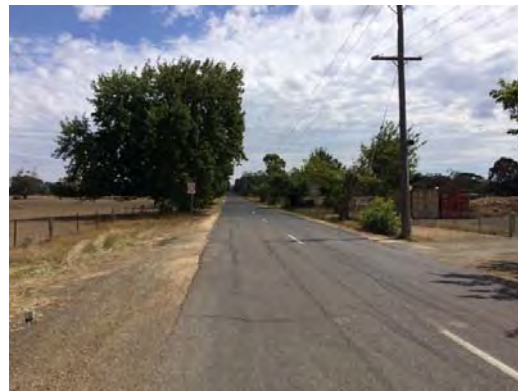
Figure 3-37: Ferrier Road (looking W)
