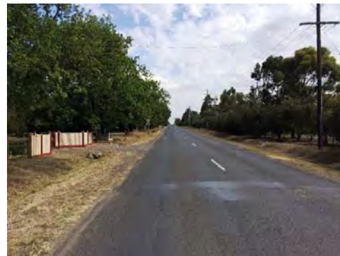
Figure 3-19: Kilmore Road (looking W)
