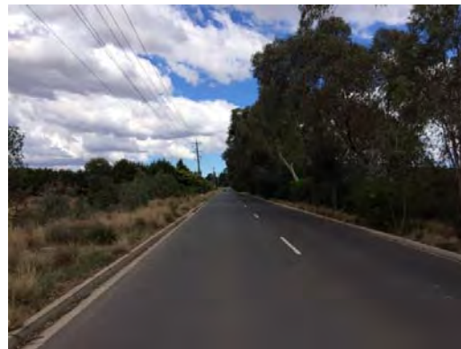
Figure 3-51: Barry Road (looking S)
