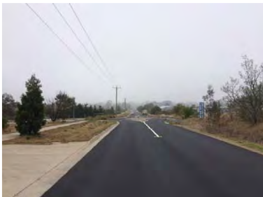
Figure 3-46: Brady Road (looking N)
