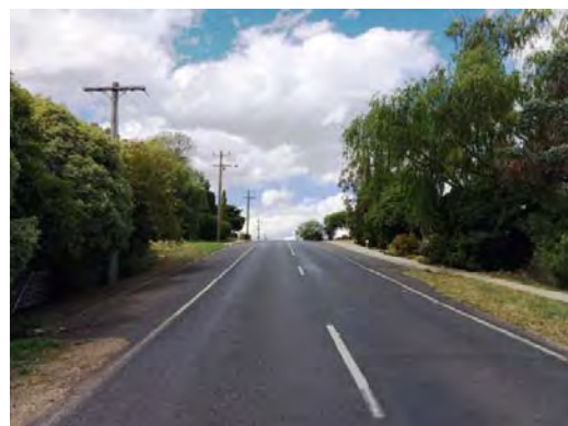
Figure 3-41: Howey Street (looking W)
