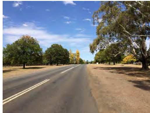
Figure 3-33: Sheedy Road (looking SE)
