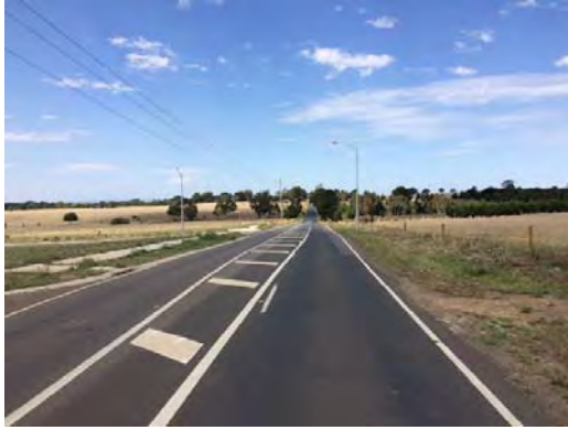
Figure 3-38: Brooking Road (looking E)
