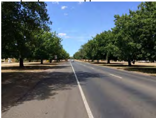
Figure 3-8: Saunders Road (looking E)
