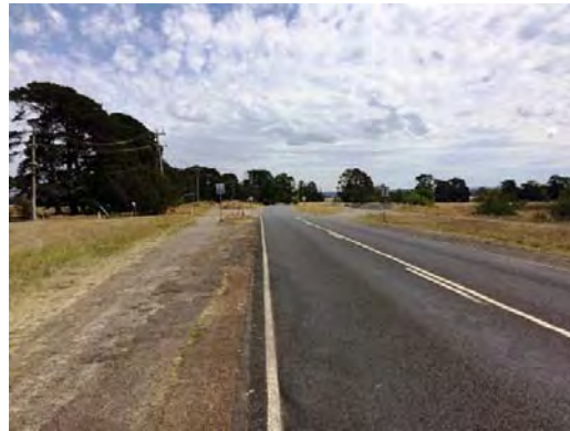
Figure 3-21: Ross Watt Road (looking W)
