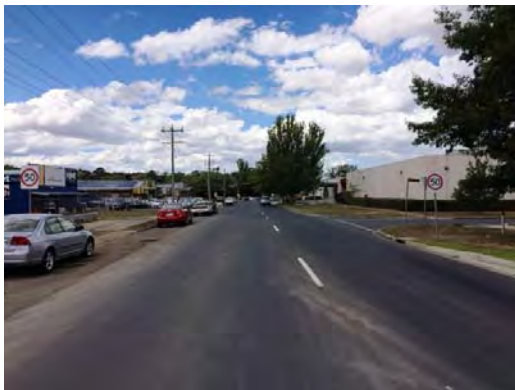
Figure 3-6: Robertson Street (looking E)
