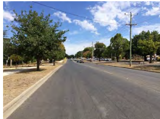
Figure 3-3G Gisborne Melton Road (looking S)
