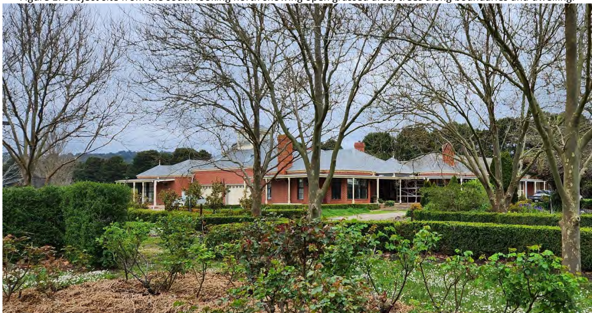
Figure 2. Brick dwelling from the south east looking northwest showing established gardens.
