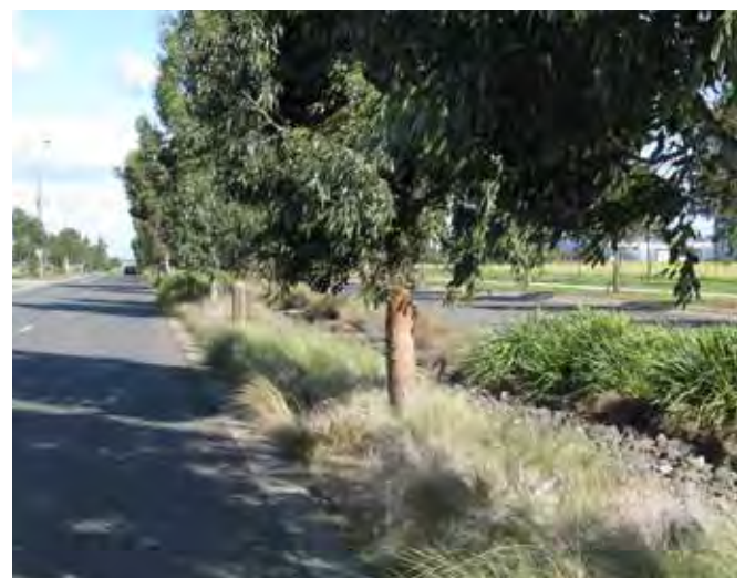
Figure 12 - Example of a swale utilised to irrigate plants and infiltrate water
