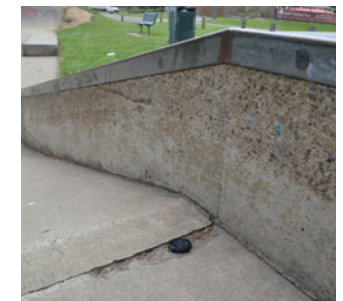
Cracking / surface damage at joints.
