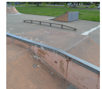
Cracking / rough surfacing on obstacles.
