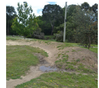
Eroded berm.
