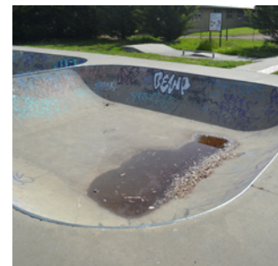
Pooling of water at base of bowl.
