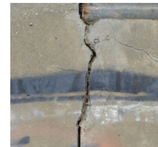
Concrete cracking at joints.
