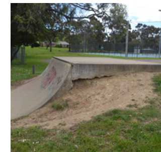
Erosion of earthworks around skatepark.
