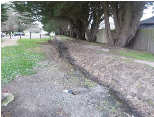
An open drain
