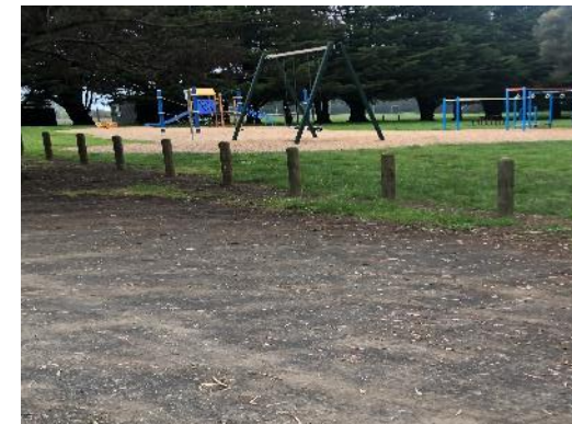
Internal bollard fencing in good condition
