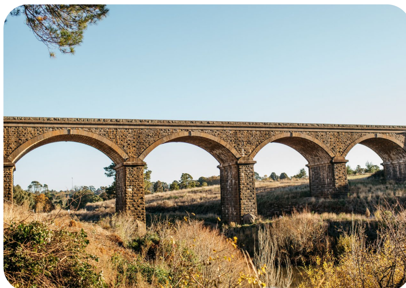
Malmsbury Viaduct, Malmsbury
