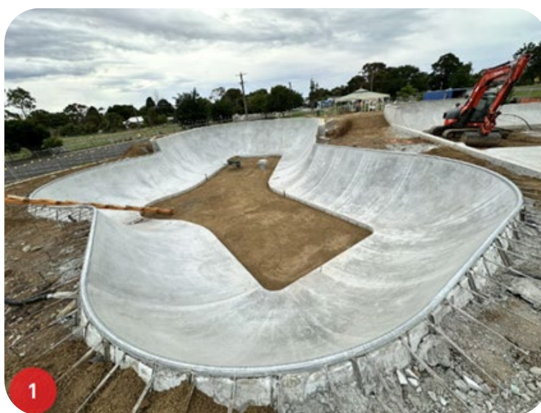
Romsey Skatepark concrete works.
