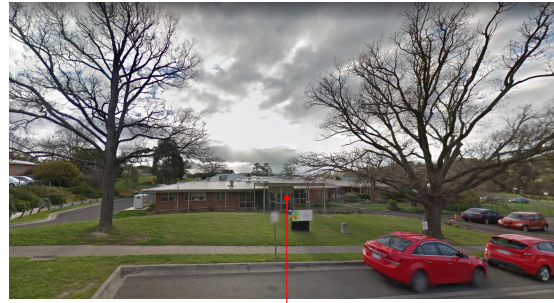
ENTRY TO GISBORNE OAKS NURSING HOME
