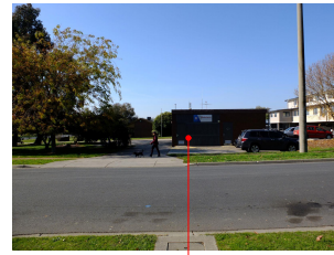
53 ROBERTSON STREET SINGLE STOREY GISBORNE AMBULANCE
