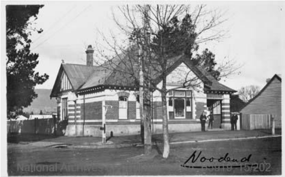
Figure 3.12 Woodend Post Office, c1905. (Source: National Archives of Australia)
