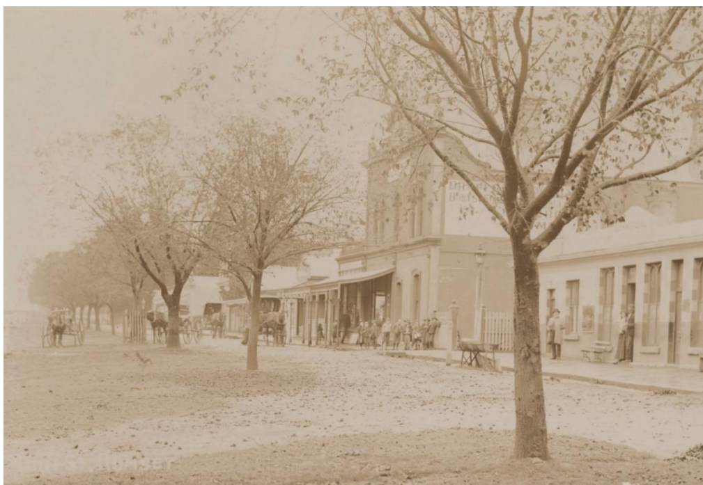
Figure 5.7 Main Street, Romsey, in 1904. (Source: State Library Victoria, Accession No. H90.140/619)
