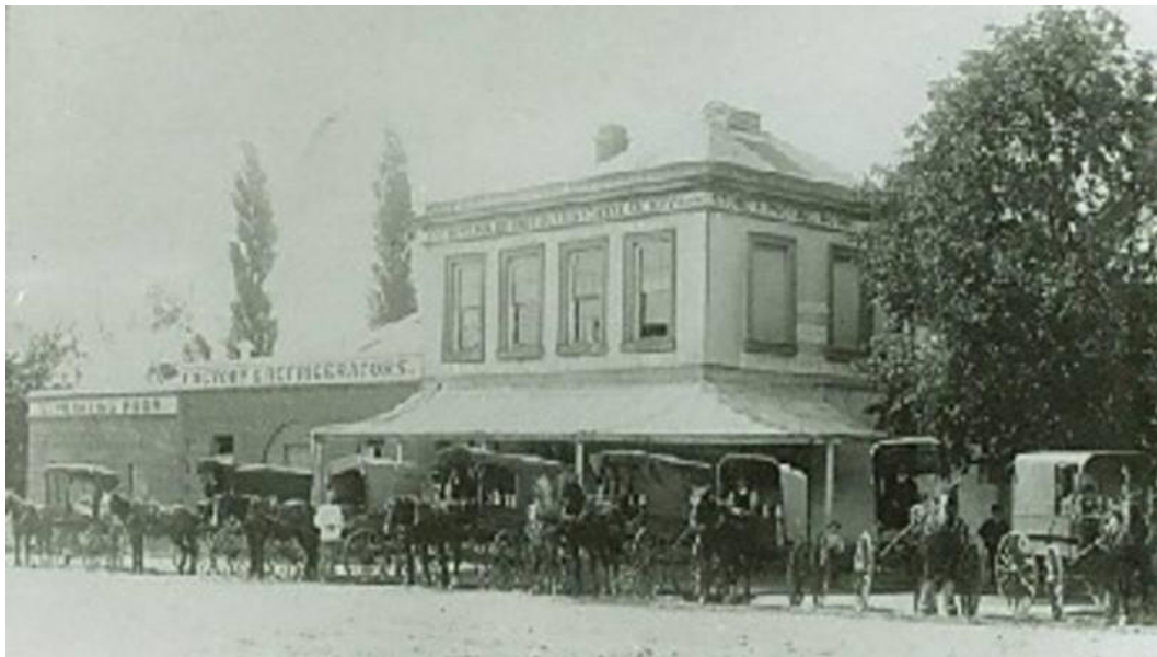
Figure 5.1 Kyneton Butter and Cheese Factory, originally built as a flour mill in the 1860s. (Source: National Trust of Australia (Vic) Register, B6387)
