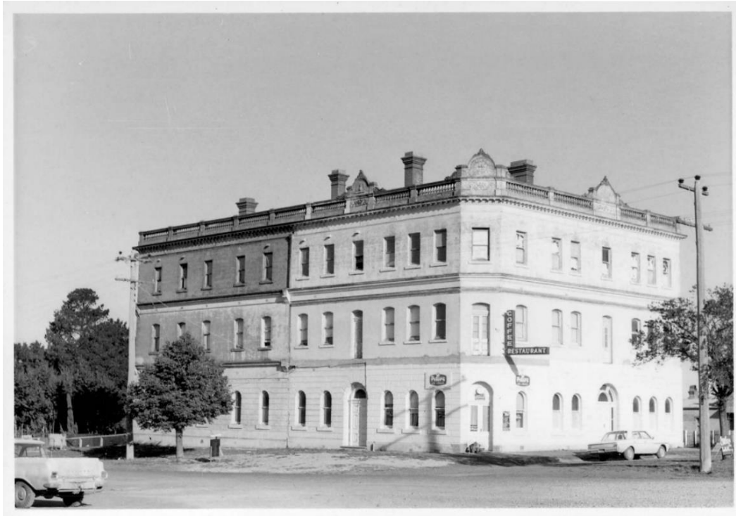
Figure 3.7 The 52-roomed Macedonia Hotel, Lancefield, built in 1889. (Source: State Library Victoria, Record ID 9939659197107636)
