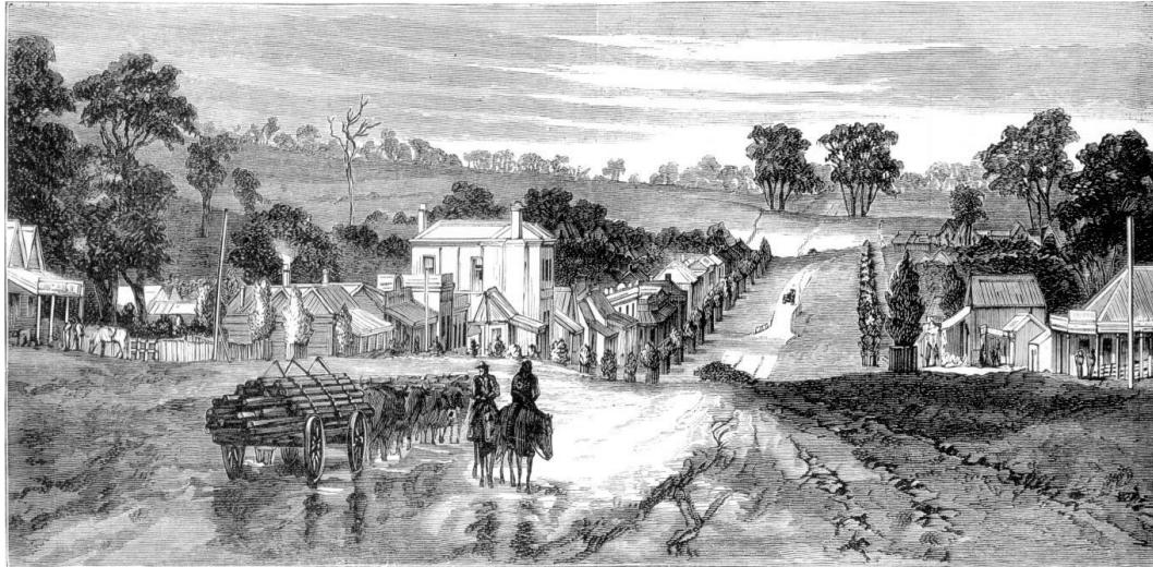
Figure 6.6 The road into Romsey, 1881. (Source: State Library Victoria, Accession No. IAN29/06/81/124a)
