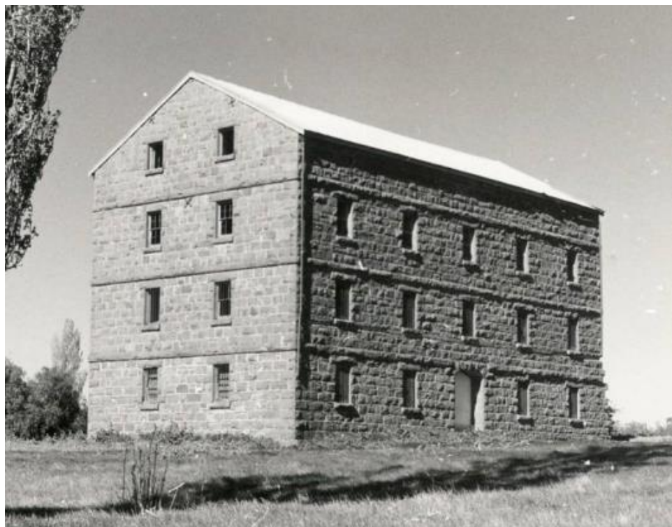
Figure 5.2 Degraves flour mill, Carlsruhe, off the Calder Highway. (Source: National Trust of Australia (Victoria) Register, B0722)
