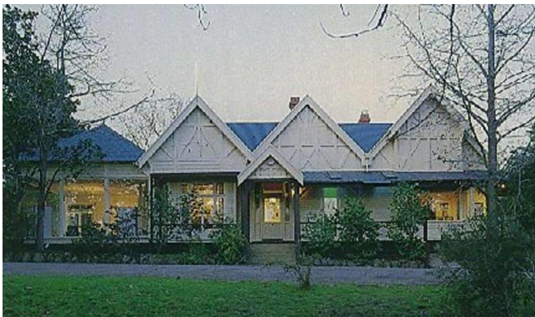
Figure 6.20 'Dromkeen', Riddells Creek built in 1889 to a design by Hyndman and Bates, for Judge Arthur Chomley. (Source: NTAV Register, B5677)
