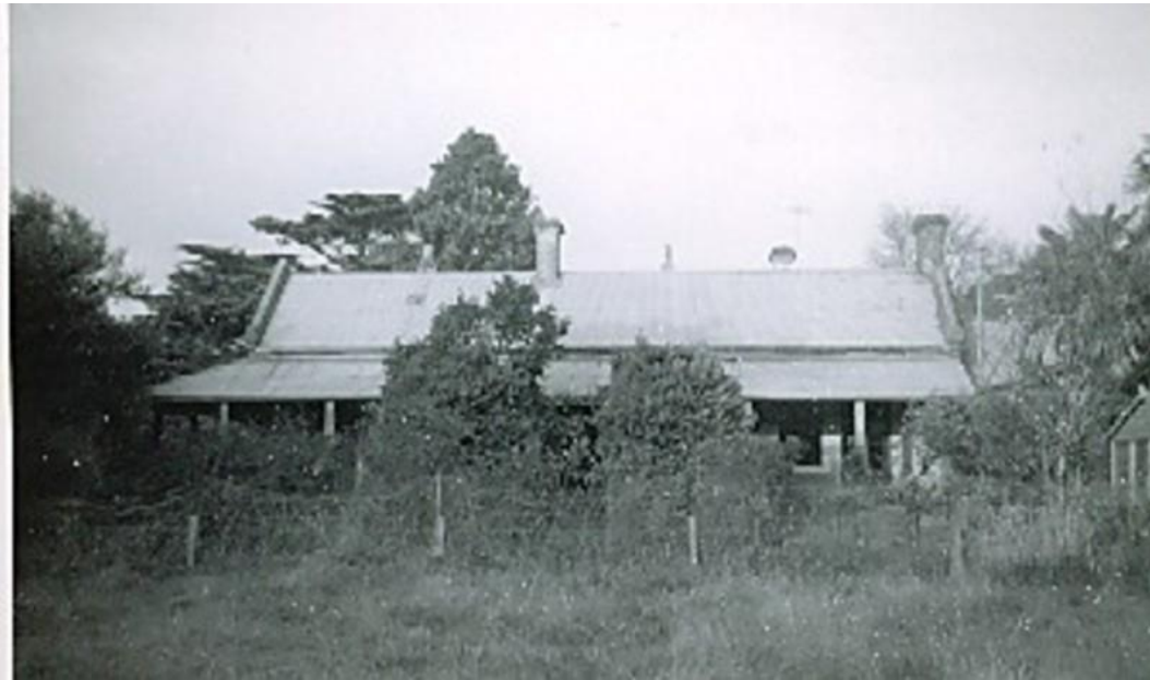
Figure 6.8 'Elderslie' homestead, New Gisborne. (Source: NTAV Register, B1652)
