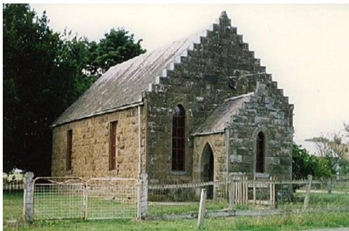
Figure 8.5 Former Newman Presbyterian Church, built in 1868. (Source: NTAV Register, B6352)
