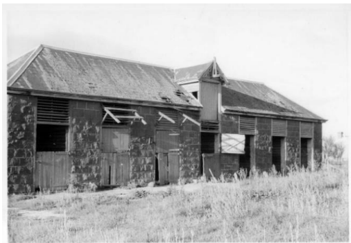
Figure 4.5 Bluestone stables, Kyneton, photographed by John T Collins in 1963. (Source: State Library Victoria, Accession No. H97.250/2022)
