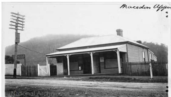
Figure 3.14 Upper Macedon (Mount Macedon) Post Office. (Source: National Archives of Australia)
