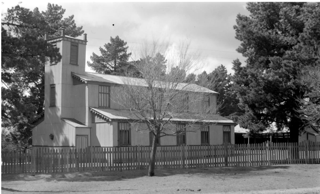
Figure 8.2 St Paul's Anglican Church, Gisborne, built from iron in 1858 (now demolished). (Source: State Library Victoria, Accession No. H32492/5898)
