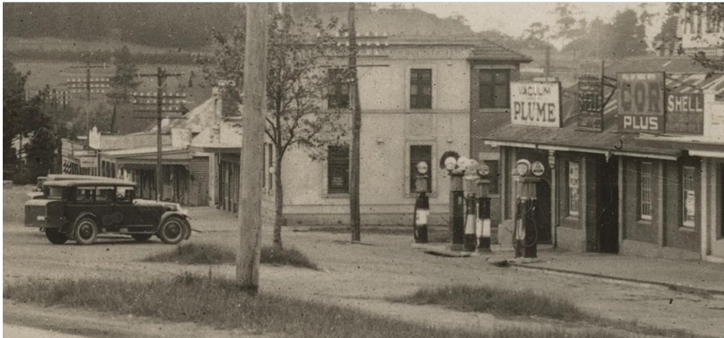
Figure 3.9 Detail of a photograph of Woodend, c1930, showing a Shell petrol station with petrol bowsers on the footpath. (Source: State Library Victoria, Record ID 9937678623607636)
