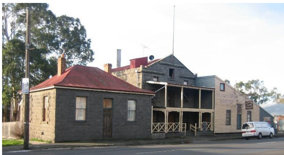
Figure 5.3 Willis' Flour Mill, Kyneton, built in 1862. (Source: Victorian Heritage Register, H2186)
