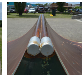
Repairs to skatepark steel.
