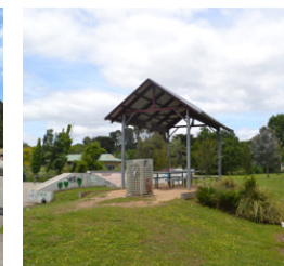
Sheltered seating area.
