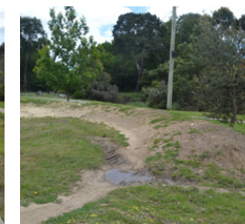
Eroded berm.
