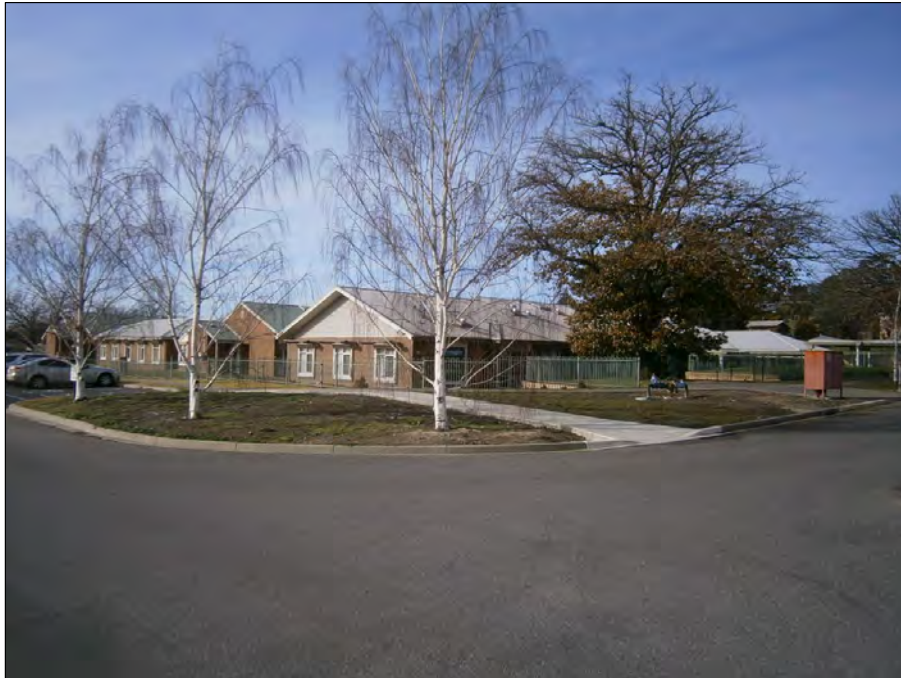
Rear of Gisborne Oaks from Robertson Street
