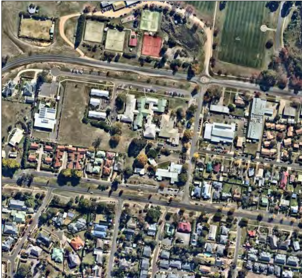
Aerial photo showing the site context
