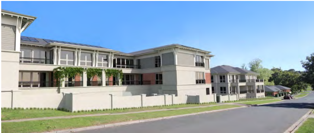
View of proposed retirement village from Neal Street looking to the north (no vegetation)
