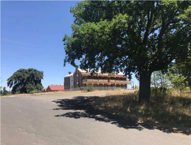
Image 1 (above) View looking southwest showing the hospital building relative to Tree 1, a Mod-B rated Weeping Wych Elm (left) and Tree 40, a High rated English Oak (right).
