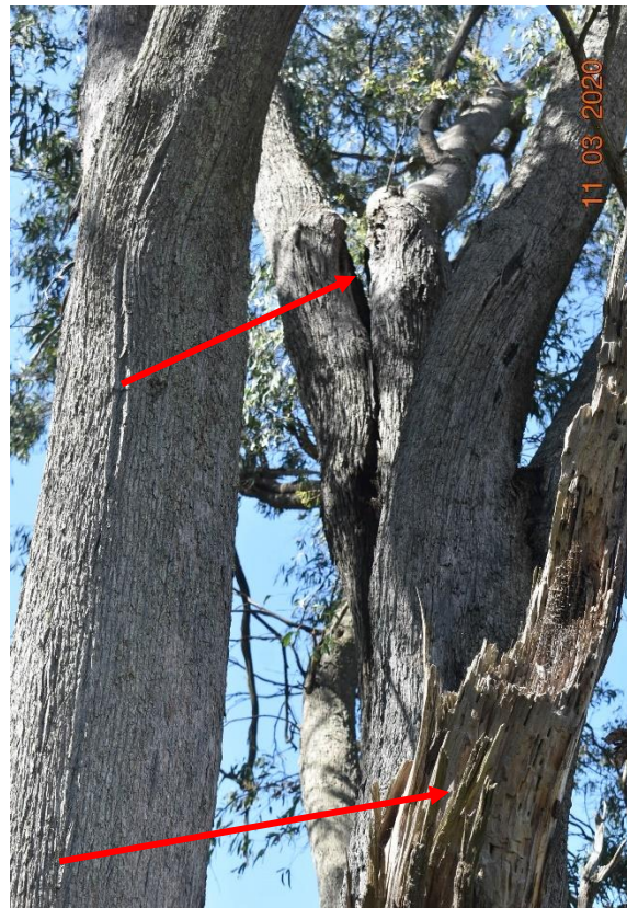
Figure 4 Tree 8 with splitting stems and recent failures following storm damage
