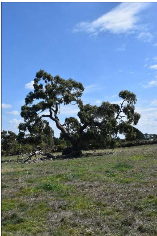
Tree #1, showing the former leading stem failed on the ground and the reformed canopy.
