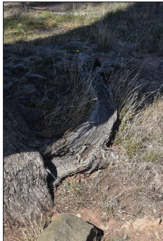
Showing one of many structural roots dead and decayed from cattle compaction and changed soil grade.
