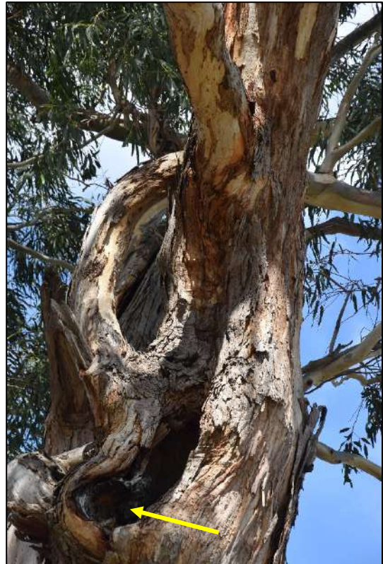
Showing the part considered most likely to fail, an area of hollowing and decay at the base of a large branch (arrow).
