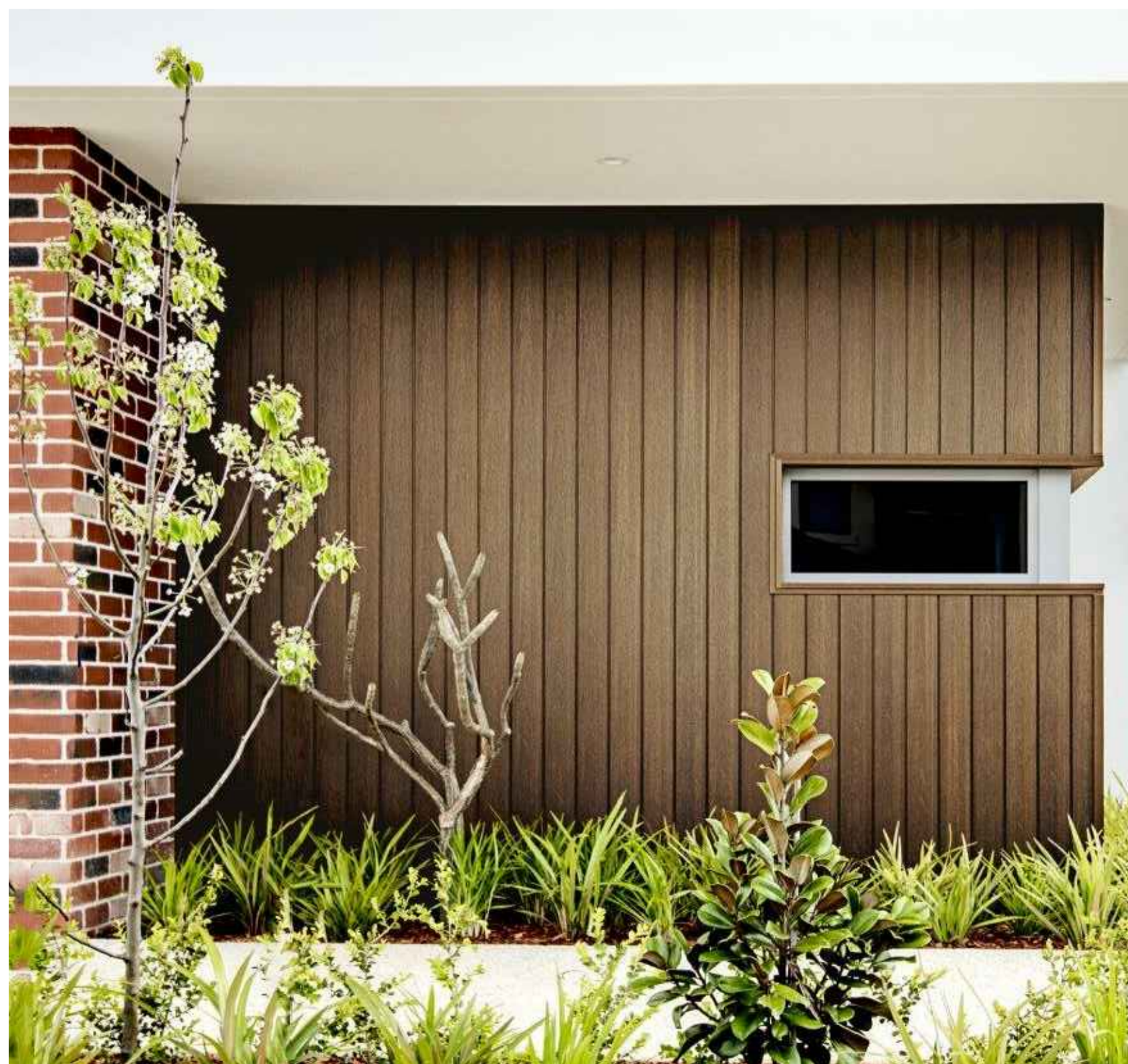
TEAK TIMBER CLADDING
