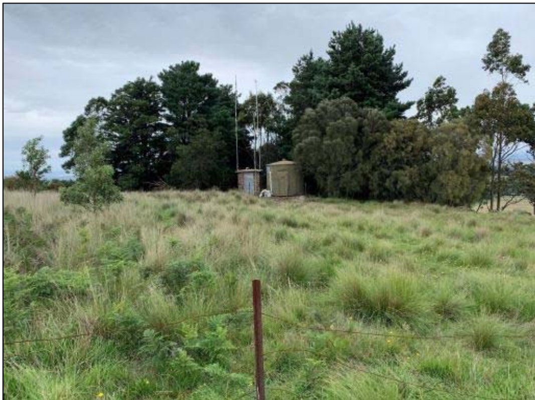
Figure 7: View of existing infrastructure on the adjacent land from the former tower site
