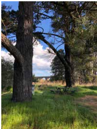
Image 43 View south toward viaduct on west bank of Coliban River
