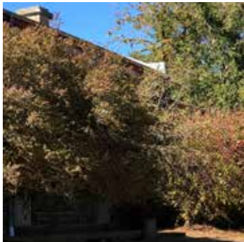
Image 31. Bluestone wall of Town Hall screened by vegetation
