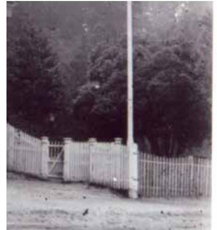
Image 49 Detail showing the c. 1913 timber gate and arrangement with adjacent timber picket fence along Mollison street.
