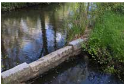
Image 64: Billabong Chain granite weir.
