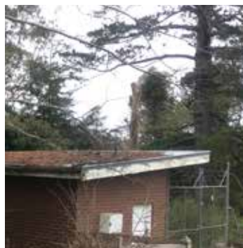
Image 26. Pump House and tank within security fencing
