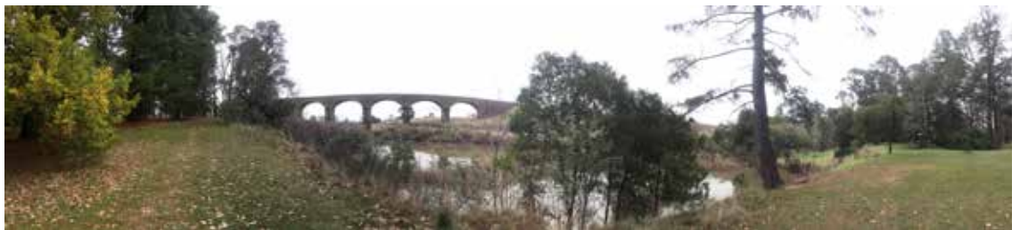
Image 59 : View toward Viaduct from the bank of the Coliban River
