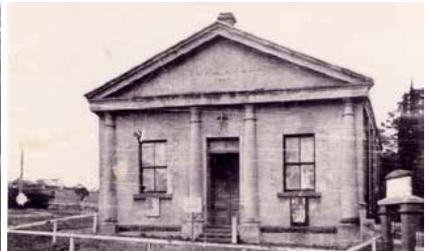
Image 47 Malmsbury Town Hall in 1949 prior to demolition of the façade. State Library of Victoria
