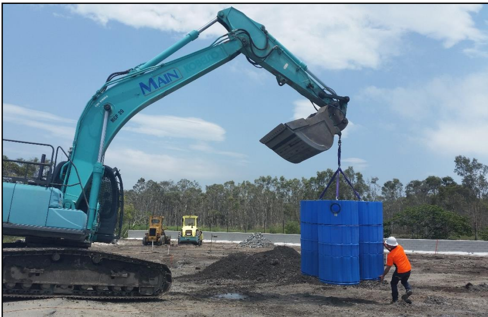
Figure 4.3: SPEL Hydrosystem (SHS.1000) installation using onsite digger
