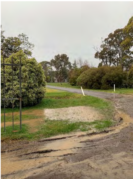
Flooding at Ligar Street – September 2019
