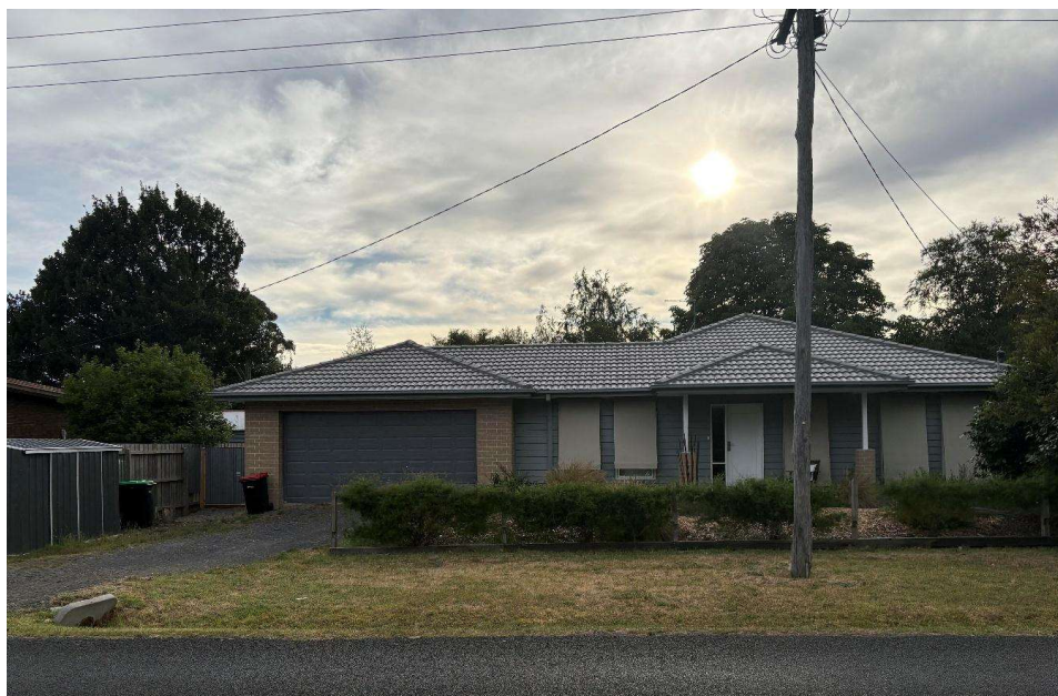
Figure 4: Image of 28 Morris Rd, west of the subject sites showing variation to side setbacks and reduced front setback under the NRZ3. January 2025.
