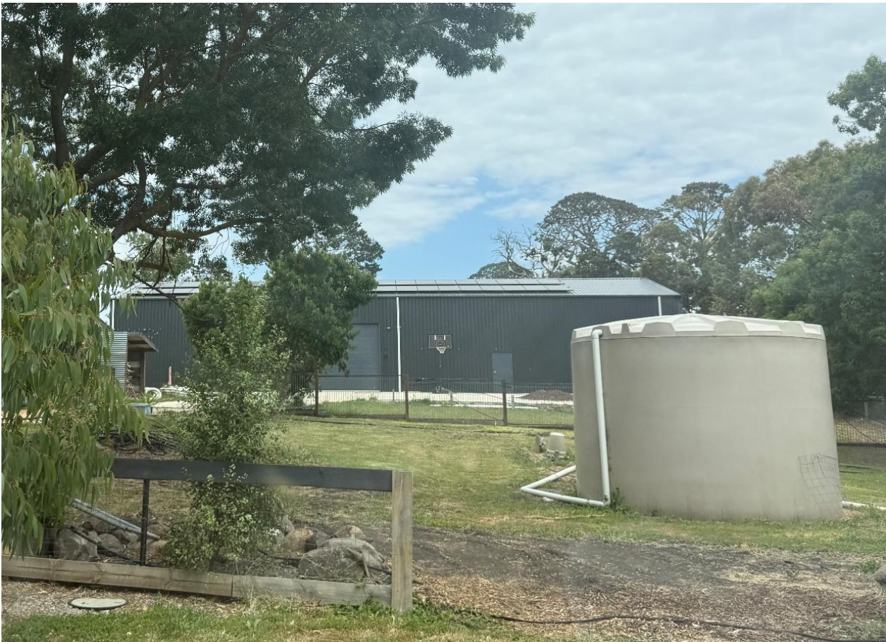
Figure 3: Outbuilding location at the rear of the site as viewed from Bolinda Darraweit Road. Note this photo was taken by the assessing officer during a site visit on 20 January 2026.
