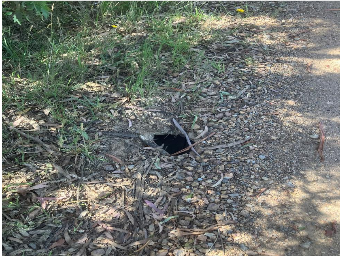
Figure 3: Broken culvert with hole on the carriageway of the Access Track section
