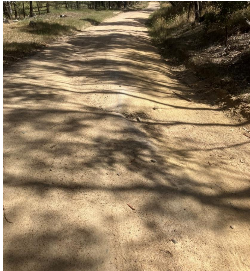
Figure 4: Overland flow path scouring road surface materials
