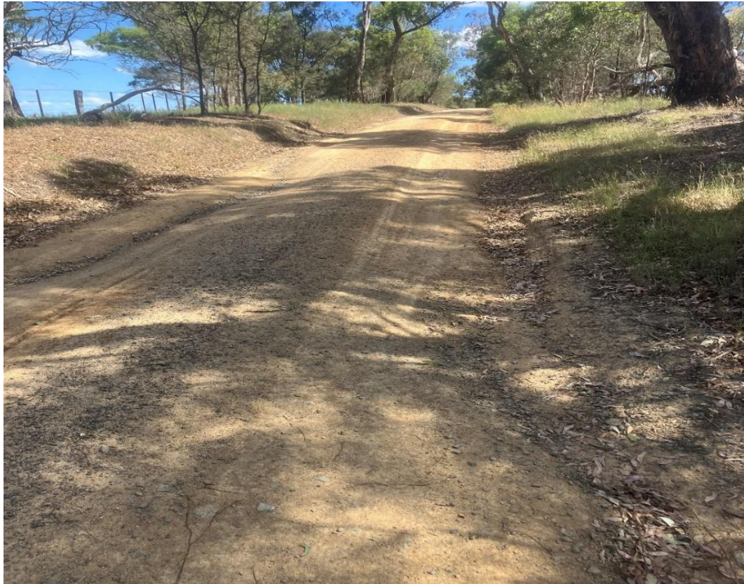
Figure 6: Overland flow path along the access track carriageway
