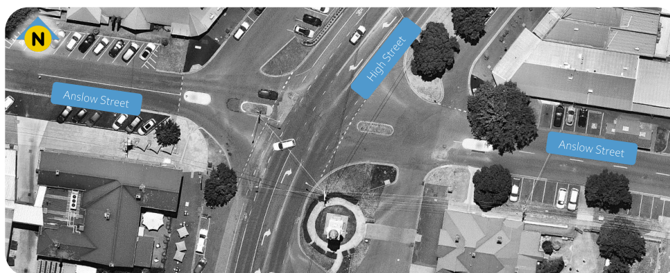
Figure 22 Anslow Street / High Street Intersection
