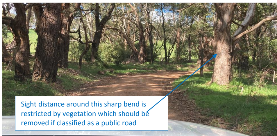
Figure 8 – Red Gap Road, Goldie illustrating trees for removal if the road widening occurs
