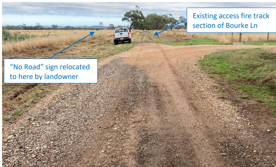
Figure 4 – Bourke Lane western end under construction
