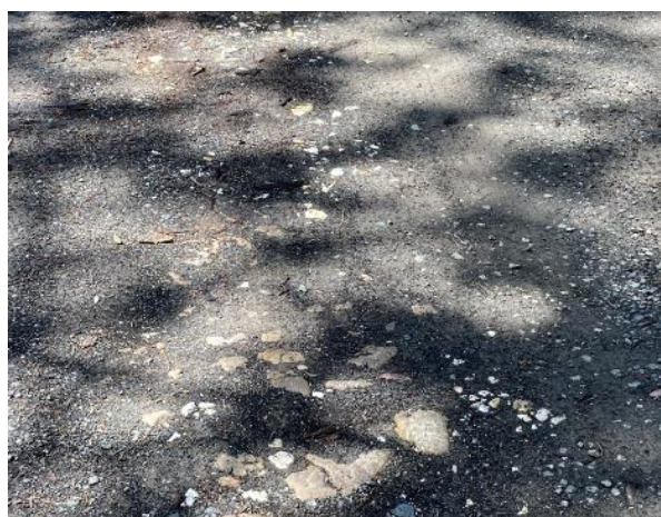
Figure 6 – Fuchsia Lane Road Surface
