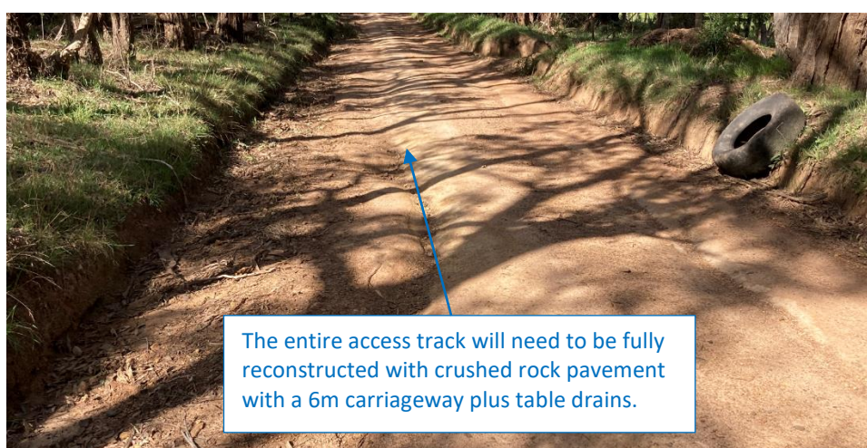
Figure 9 – Red Gap Road, Goldie illustrating compacted earth carriageway
