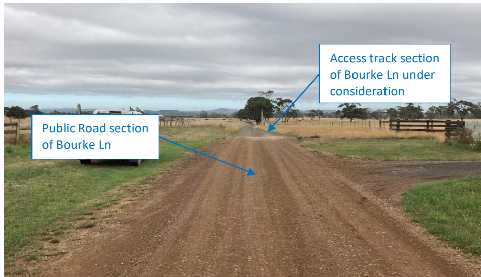
Figure 2 – Bourke Lane looking west adjacent 167 Bourke Lane
