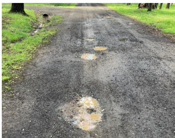
Figure 7 – Fuchsia Lane Road Surface
