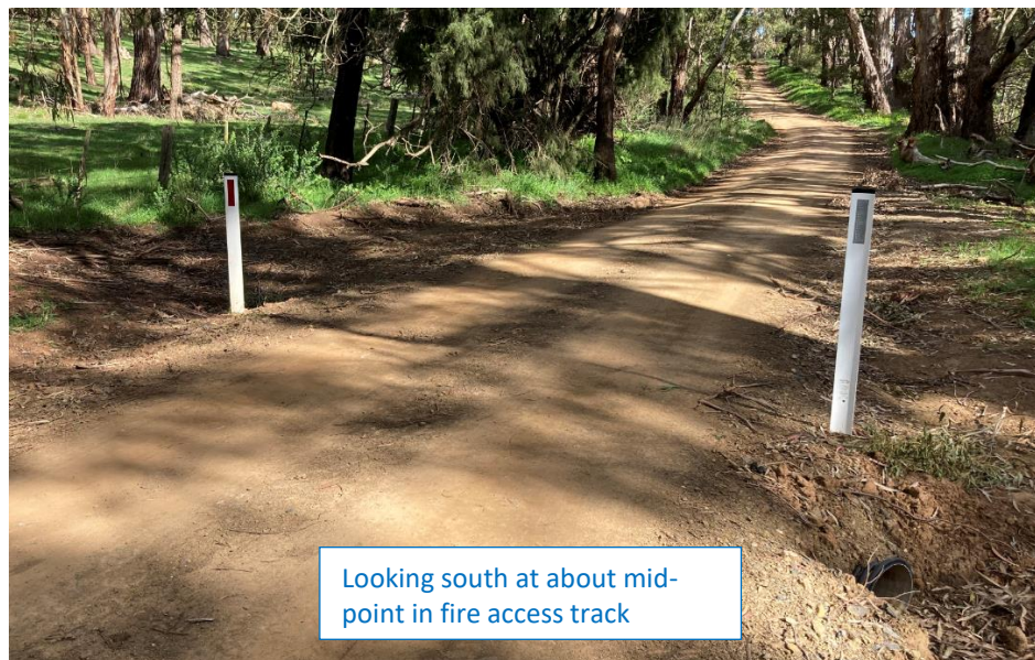
Figure 3 – Red Gap Road, Goldie looking south on the Fire Access Track
