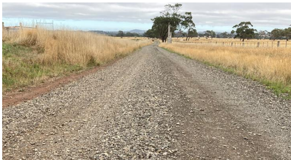
Figure 3 – Bourke Lane looking west at the mid-point (under construction)
