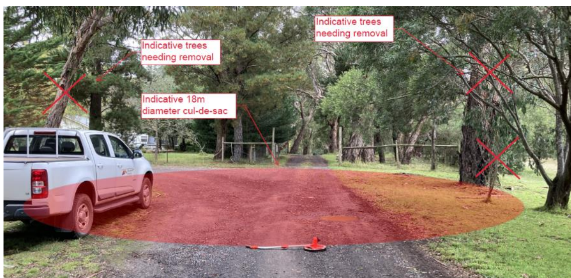
Figure 8 – Fuchsia Lane, overlay of turning circle
