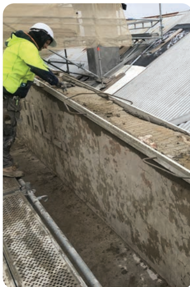
Kyneton Town Hall Façade upgrade works – repairs to render, before and after
