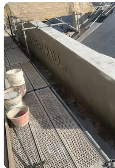
Kyneton Town Hall Façade upgrade works – repairs to render, before and after
