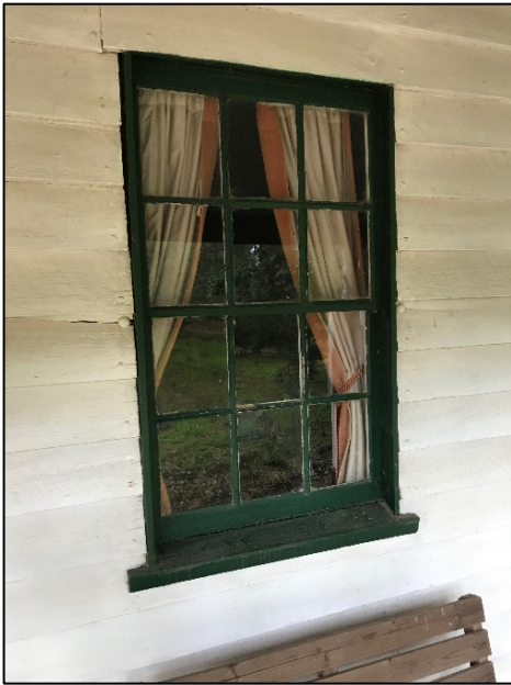
Figure 7. Detail of front multi-paned window (GJM Heritage July 2019).
