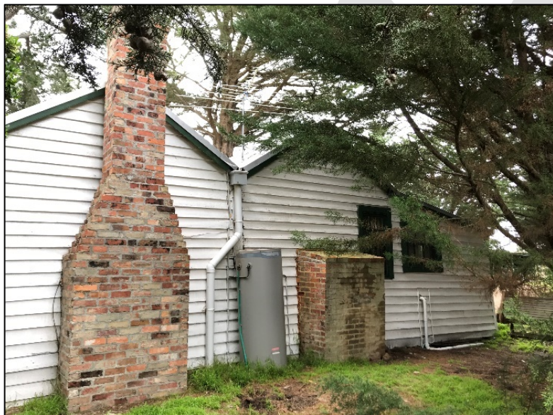
Figure 6. East elevation showing double gabled roof, brick chimney and base of removed chimney (GJM Heritage July 2019).
