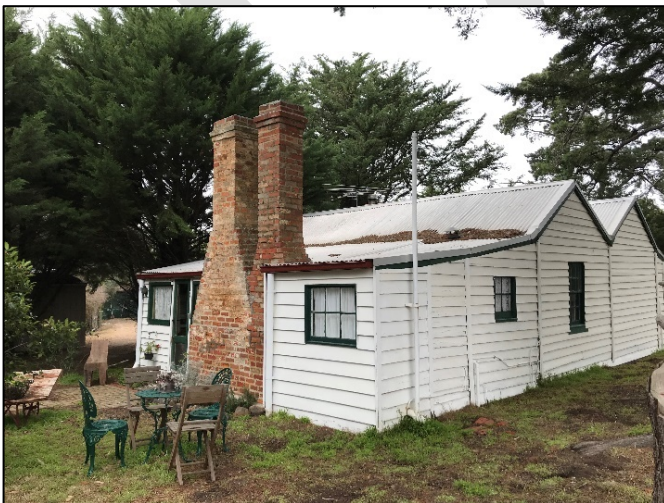
Figure 9. Rear elevation form north-west (GJM Heritage July 2019).
