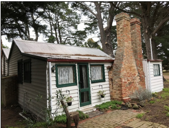
Figure 8. Rear elevation showing lean-to and double chimney stacks (GJM Heritage July 2019).
