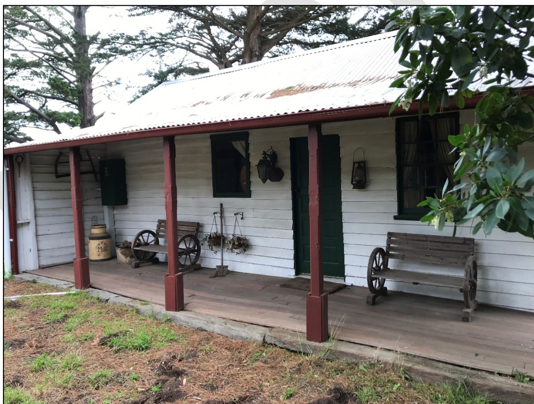
Figure 1. 111 Saunders Road, New Gisborne (GJM Heritage, 17 July 2019)
