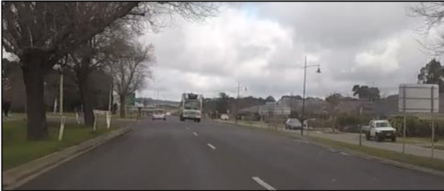
Figure 3-12 Station Road Southbound Towards Saunders Road
