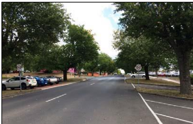
Figure 3-19 Hamilton Street Westbound from Brantome Street
