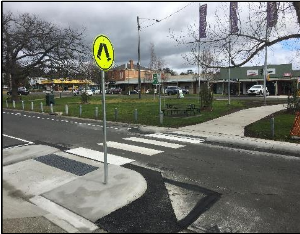
Figure 3-29 New Pedestrian Crossing on Aitken St
